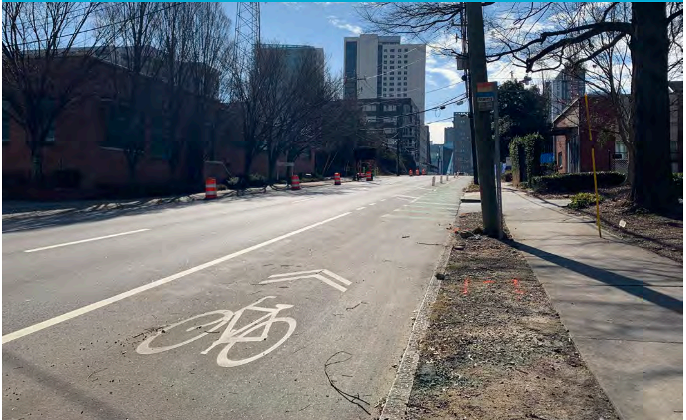
Photo of Bus Stop #4 (Looking South)
