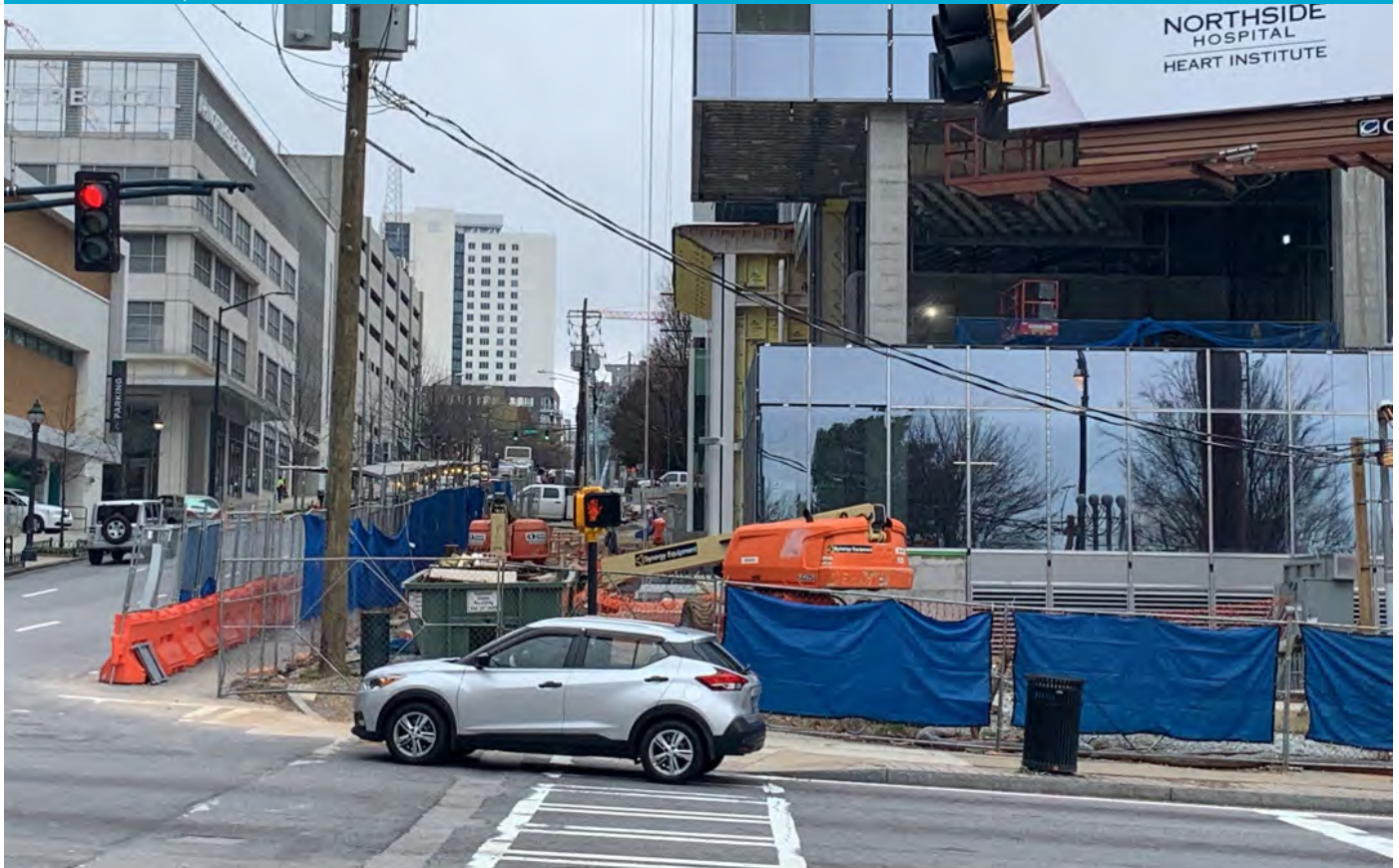
Photo of Bus Stop #3 (Looking South)
