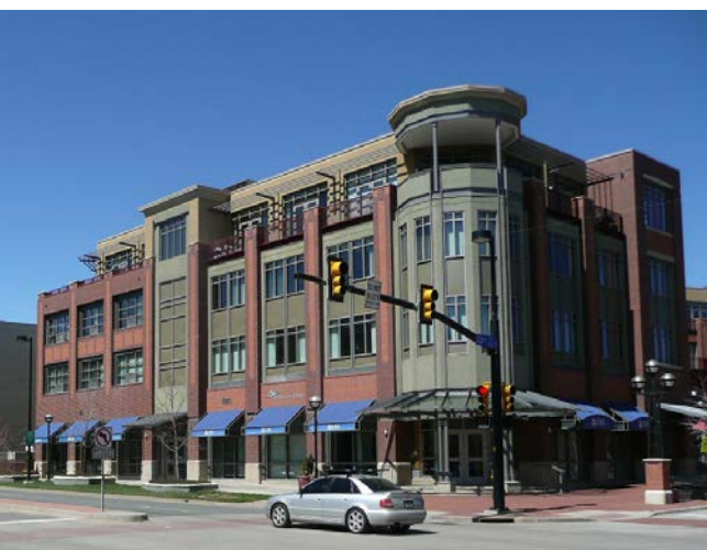
Examples of mixed use development in Boulder, CO
