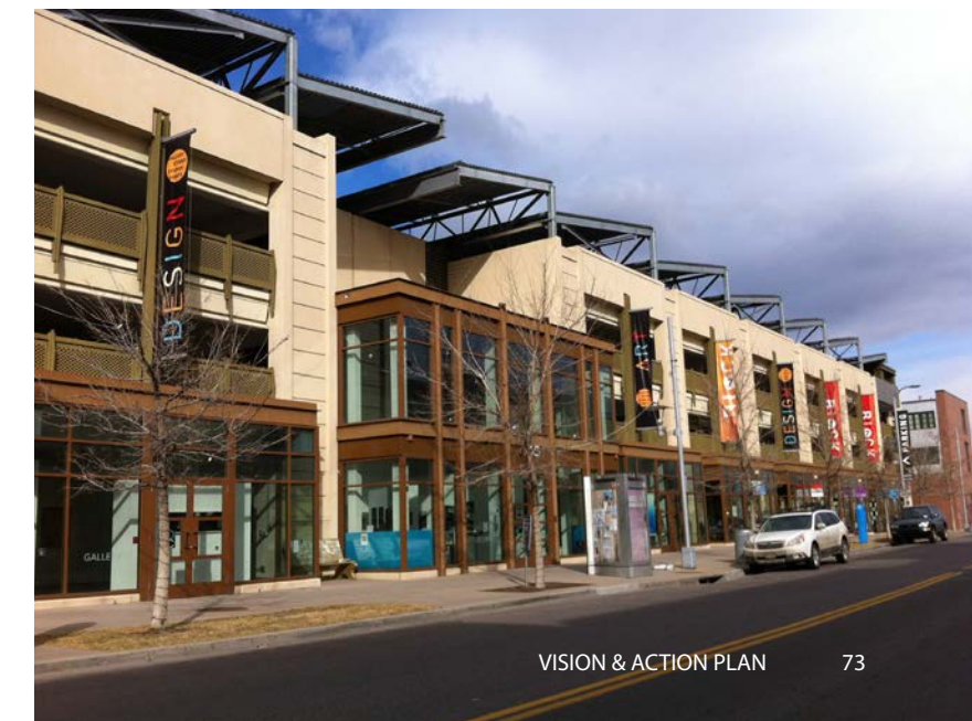
Parking structure with ground floor retail and roof top solar panels in Lakewood, CO
