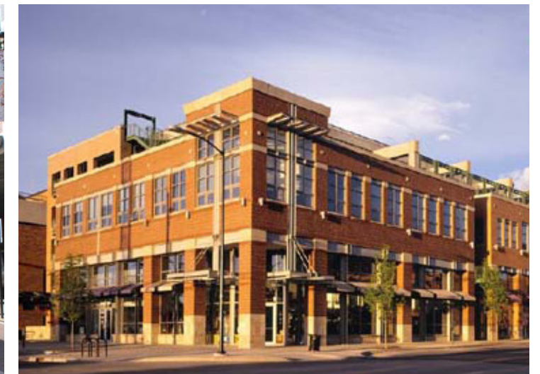
Parking areas should be screened from public view. When facing a public street, design the edges with active building uses, when feasible, or design to look like a building with similar bay rhythm and materiality. When facing an alley, use creative screening techniques, such as mesh, screens, green walls, or design to look like a building.
