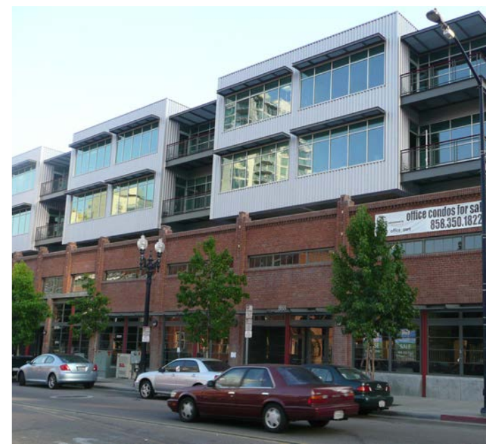
Historic office building with 2 stories of new residential development above in San Diego, CA
