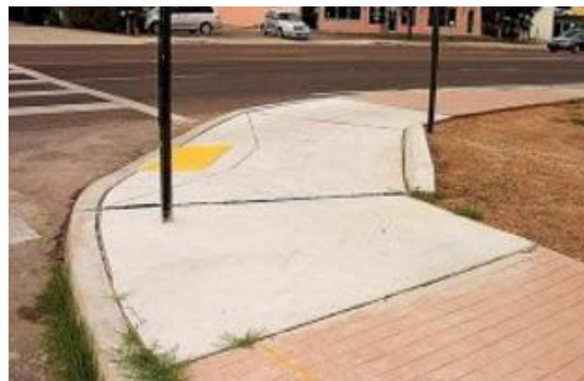
Curb ramp upgrades
