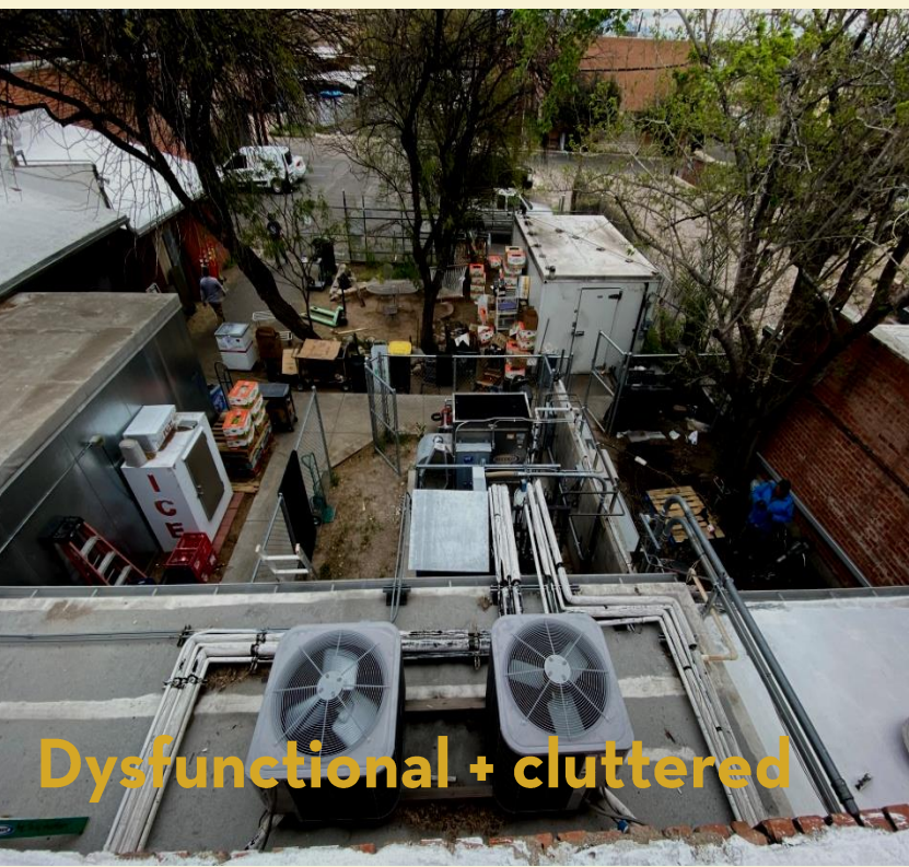
Existing Co-op Site
