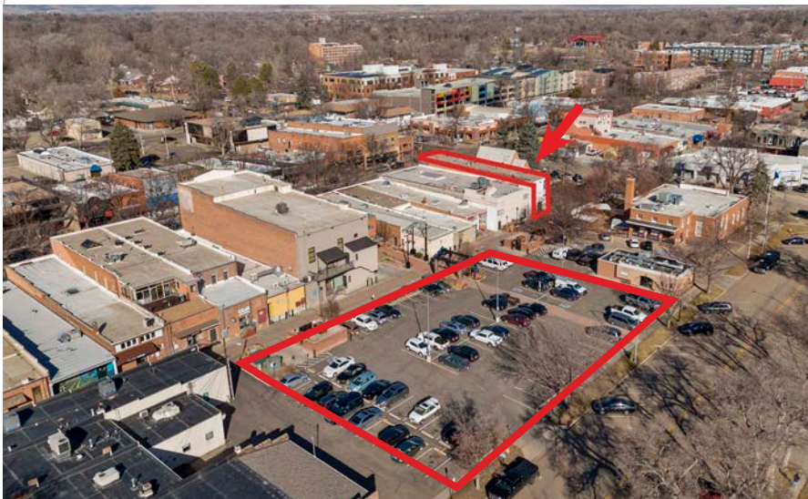
Parking for Tenants (Open, Non-Designated)
