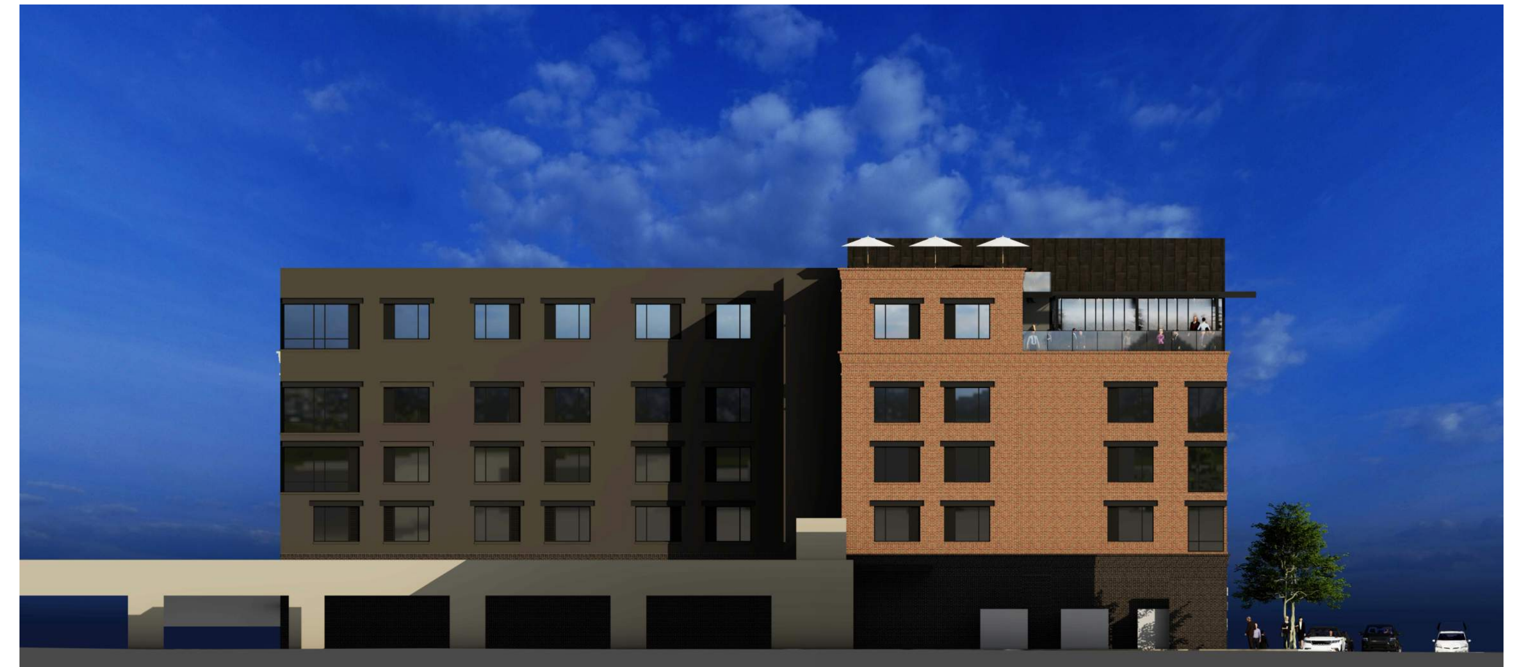
WEST: VIEW FROM ALLEY
