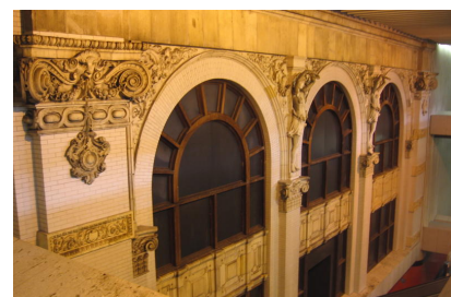
Eiseman building facade, Five Points Image via AtlantaTimeMachine / Jeff Morrison
