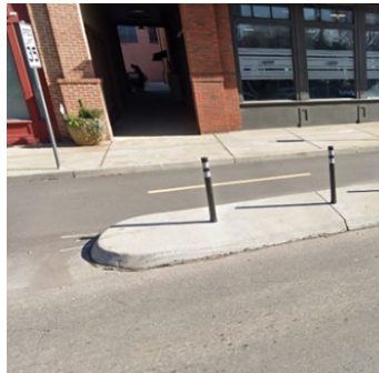
Modular Concrete Median
