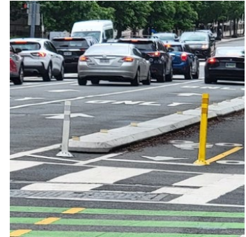
Cast-in-Place (Integral) Median
