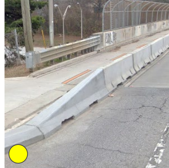
Concrete Barrier Wall
