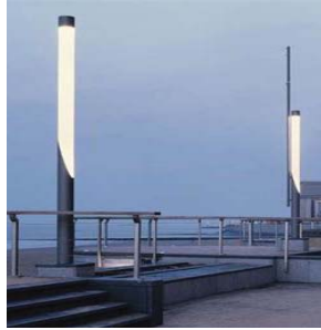
Hees Column Lighting
