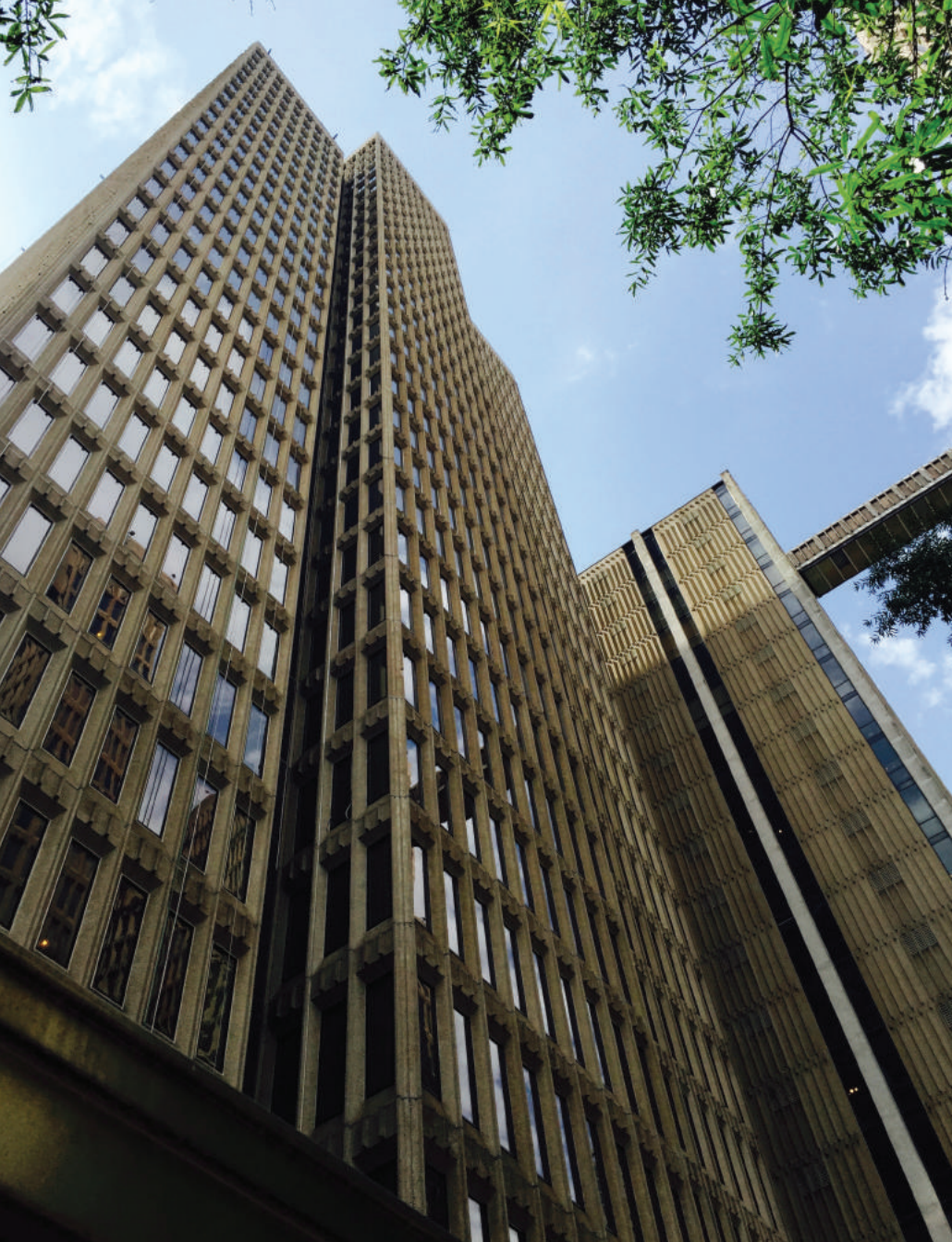
The 230 Peachtree Building (Left) and Atlanta Merchandise Mart (Right). Source: Baker, 2015.
