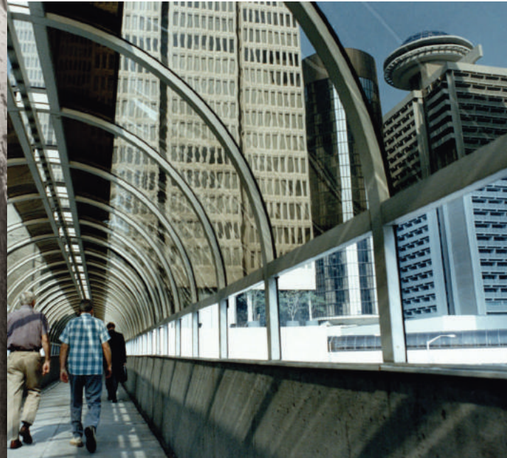
(Below) Portman used pedestrian sky bridges high above the street to provide access between various Peachtree Center buildings. Source: Atlanta Journal-Constitution Photographic Archives. Special Collections and Archives, Georgia State University Library.
