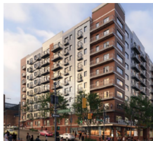
Trinity Central Flats Credit: SSOE/Stevens & Wilkinson
