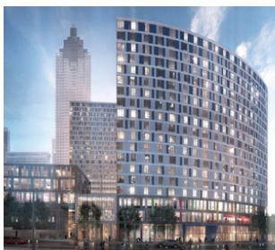
Atlanta First United Methodist Church Redevelopment
