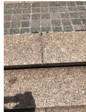
Photo 3 – Grouting of tile
