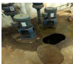
Photo 12 – Lower Pump Room
