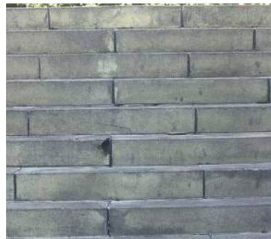
Photo 14 – Caulking of fountain steps
