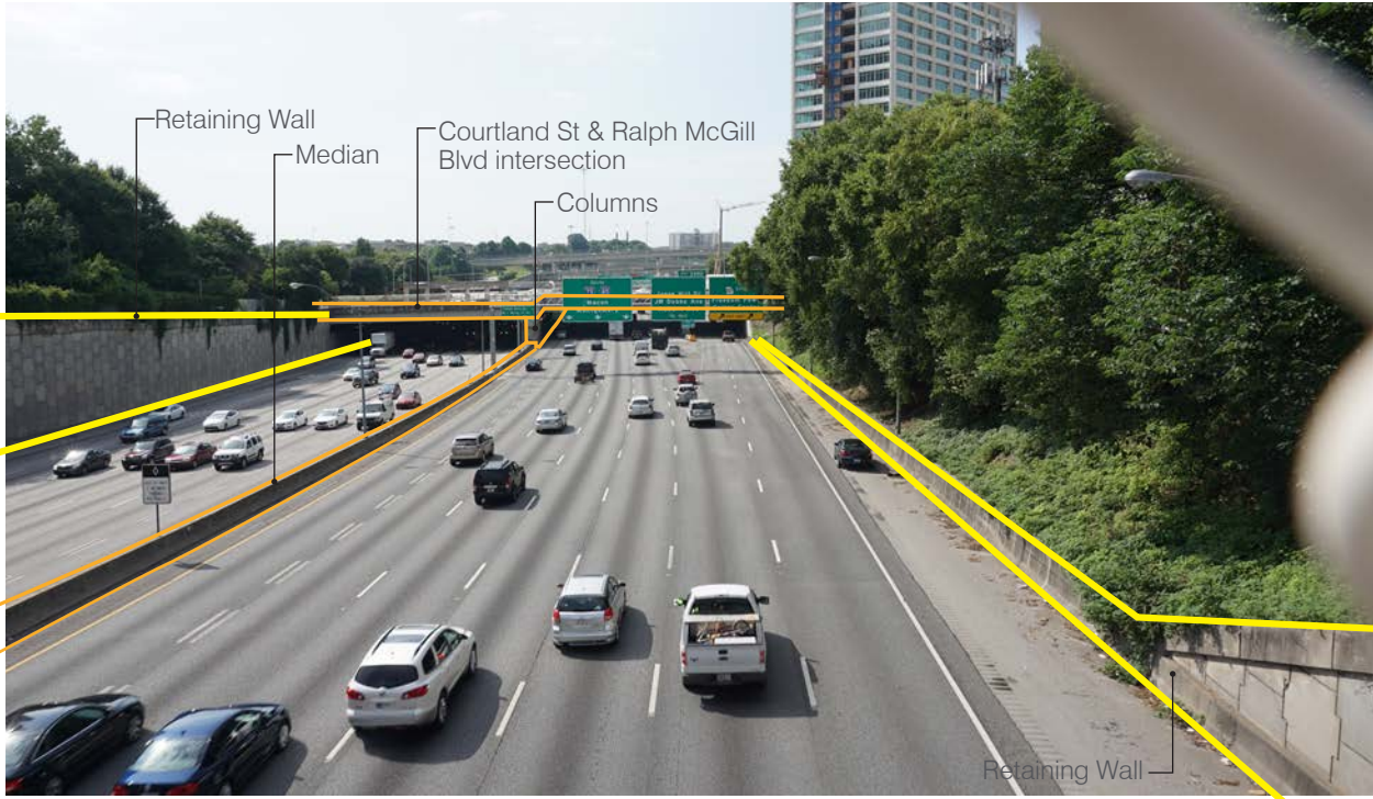
Interstate at Piedmont Ave & Baker St intersection (northeast)
