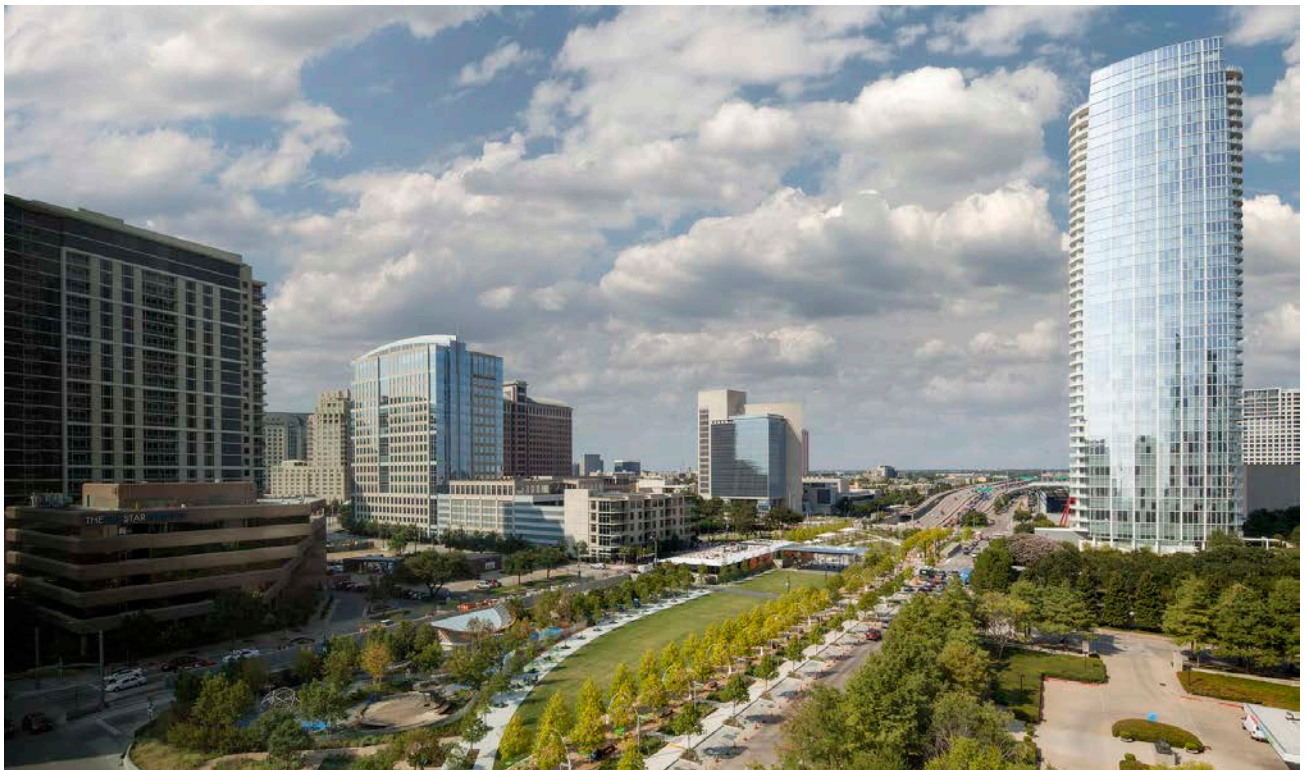
Klyde Warren Park unifies and activates a previously divided area in Dallas, Texas
