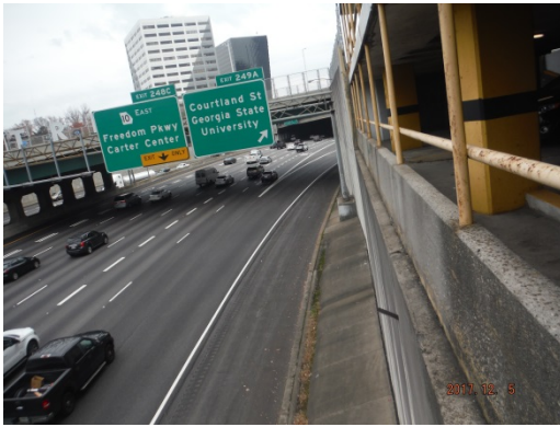
Figure A-1: Existing Wall Adjacent to Wall F
