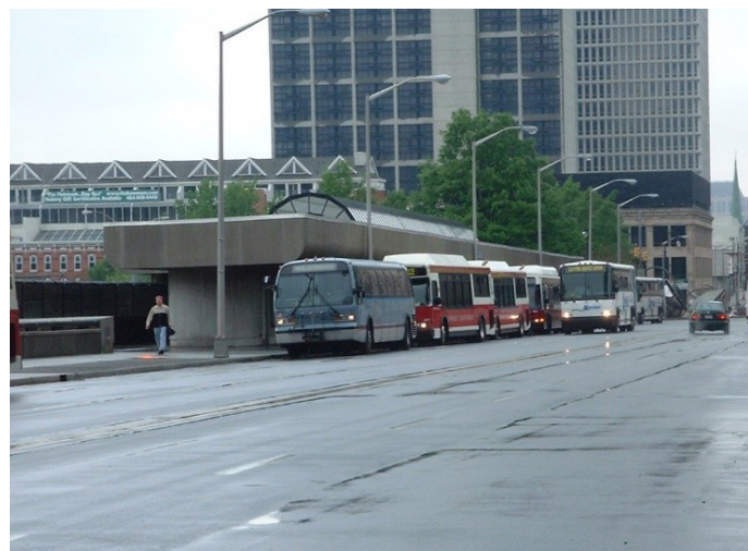
FIGURE 9. Buses Staging at Civic Center MARTA Station. 43 busses per hour stage during the peak period without a dedicated bus facility.
