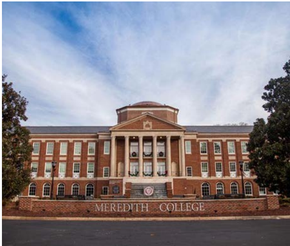
Johnson Hall Renovations
