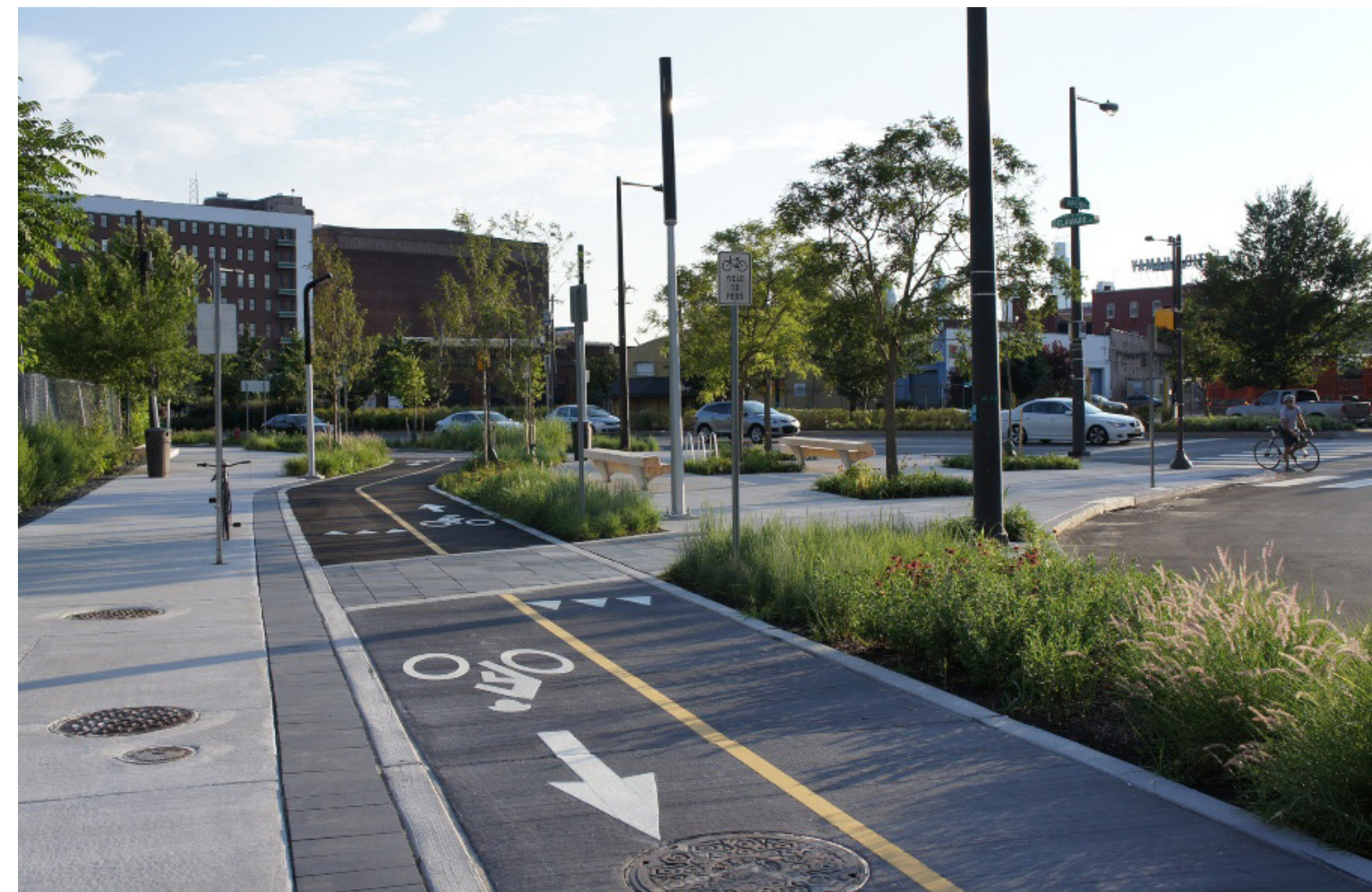
Fig. 22 | The Penn Street Trail two-way protected bike lane | Photo courtesy of NV5
