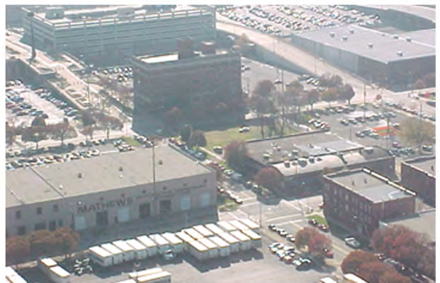
E8 - Looking southwest with intersection of Brady Street and Boston Avenue in foreground and Brady Lofts and Williams Communications in background.
