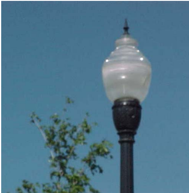
EXHIBIT 18 - TYPICAL EXAMPLE OF ORNAMENTAL PEDESTRIAN LAMP POST GLOBE-FIXTURE
