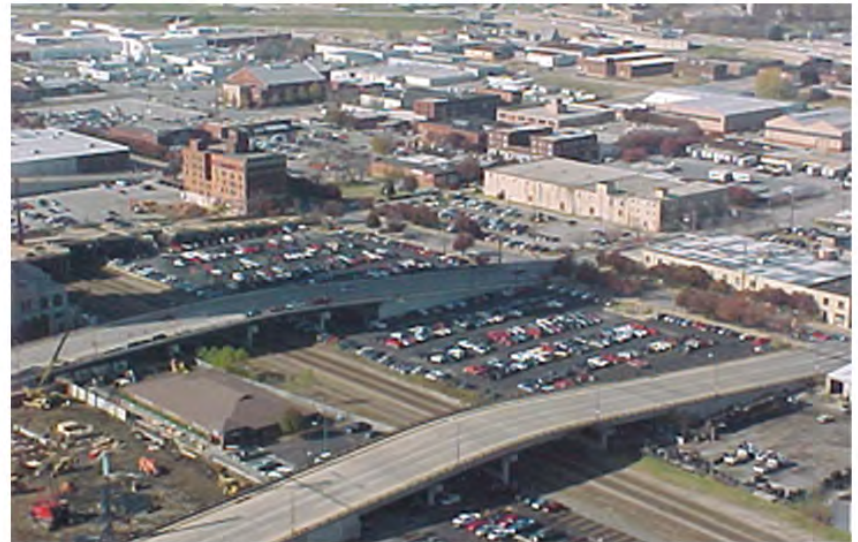
E2 - Looking west-northwest towards I-244 from Detroit Avenue Bridge.
