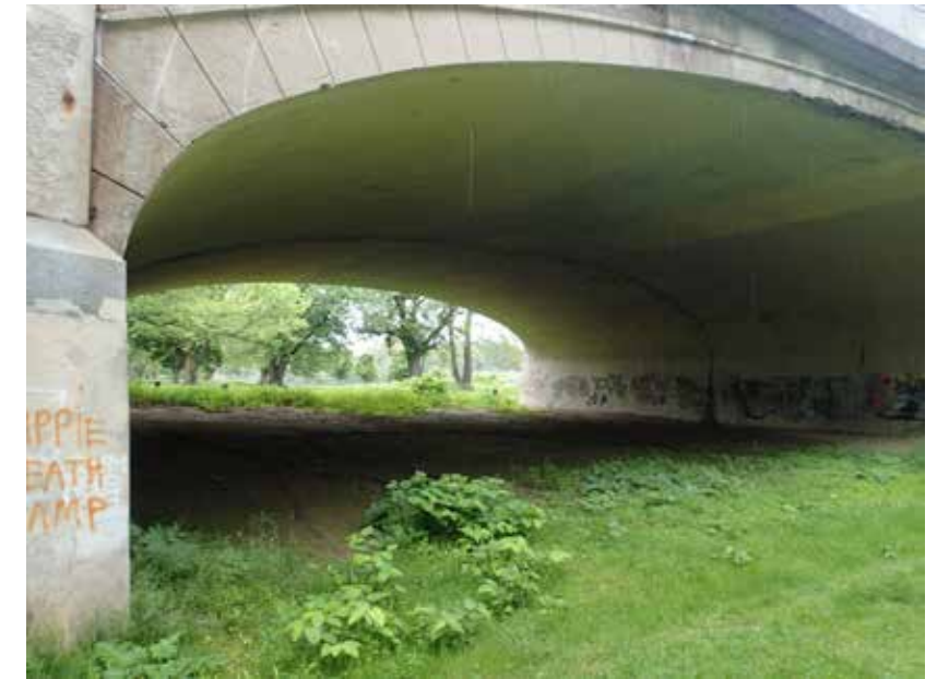
Current condition: Unused open space under Market St. bridge.
