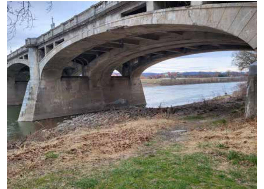
Current condition: First bridge bay over water. Includes natural protection from strong currents.
