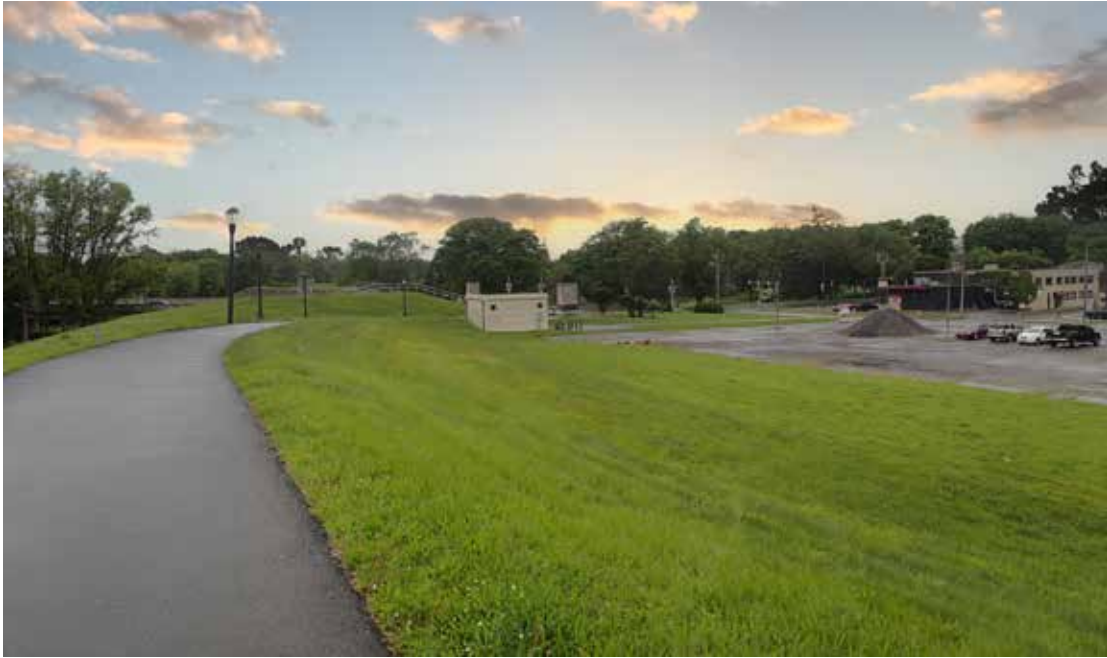
Current condition: View from levee facing south towards Market St.
