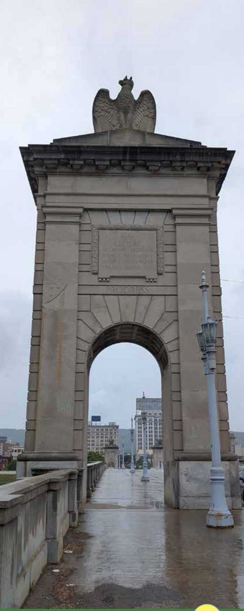
Right: Market Street Bridge looking toward downtown Wilkes-Barre
