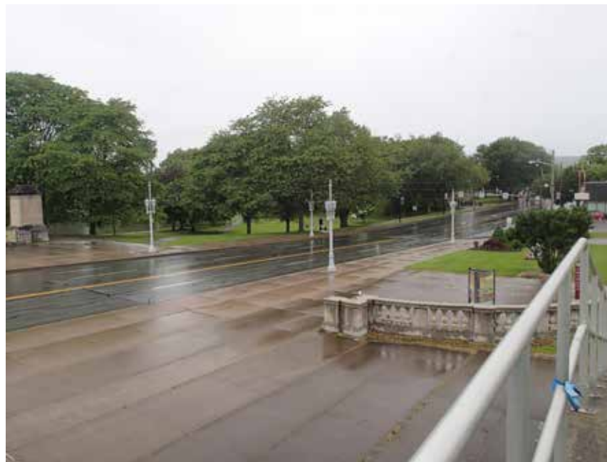
Current condition: Market St. Bridge entrance.
