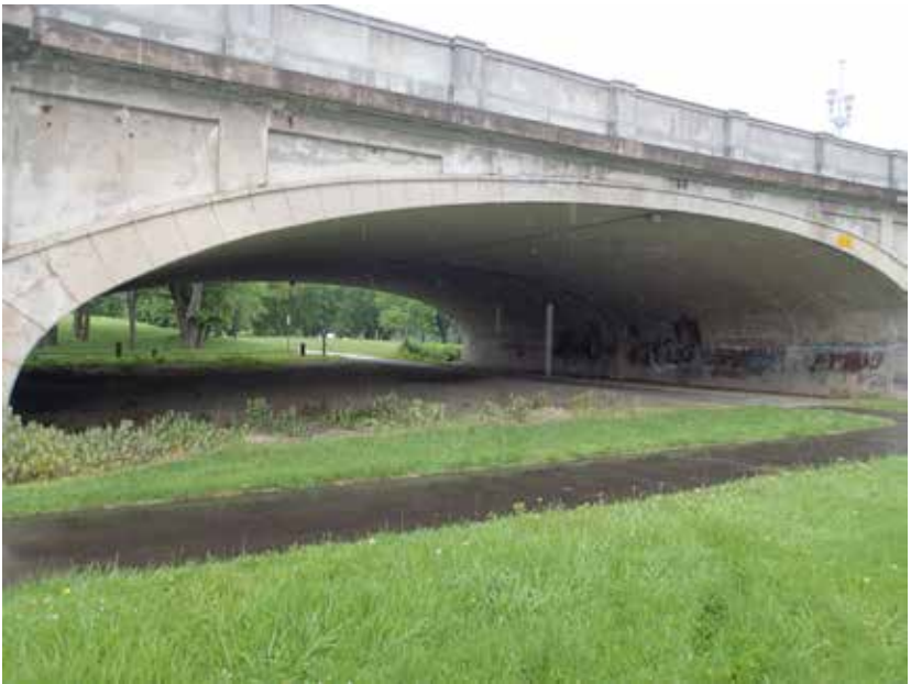
Current condition: Unused open space under Market St. Bridge.
