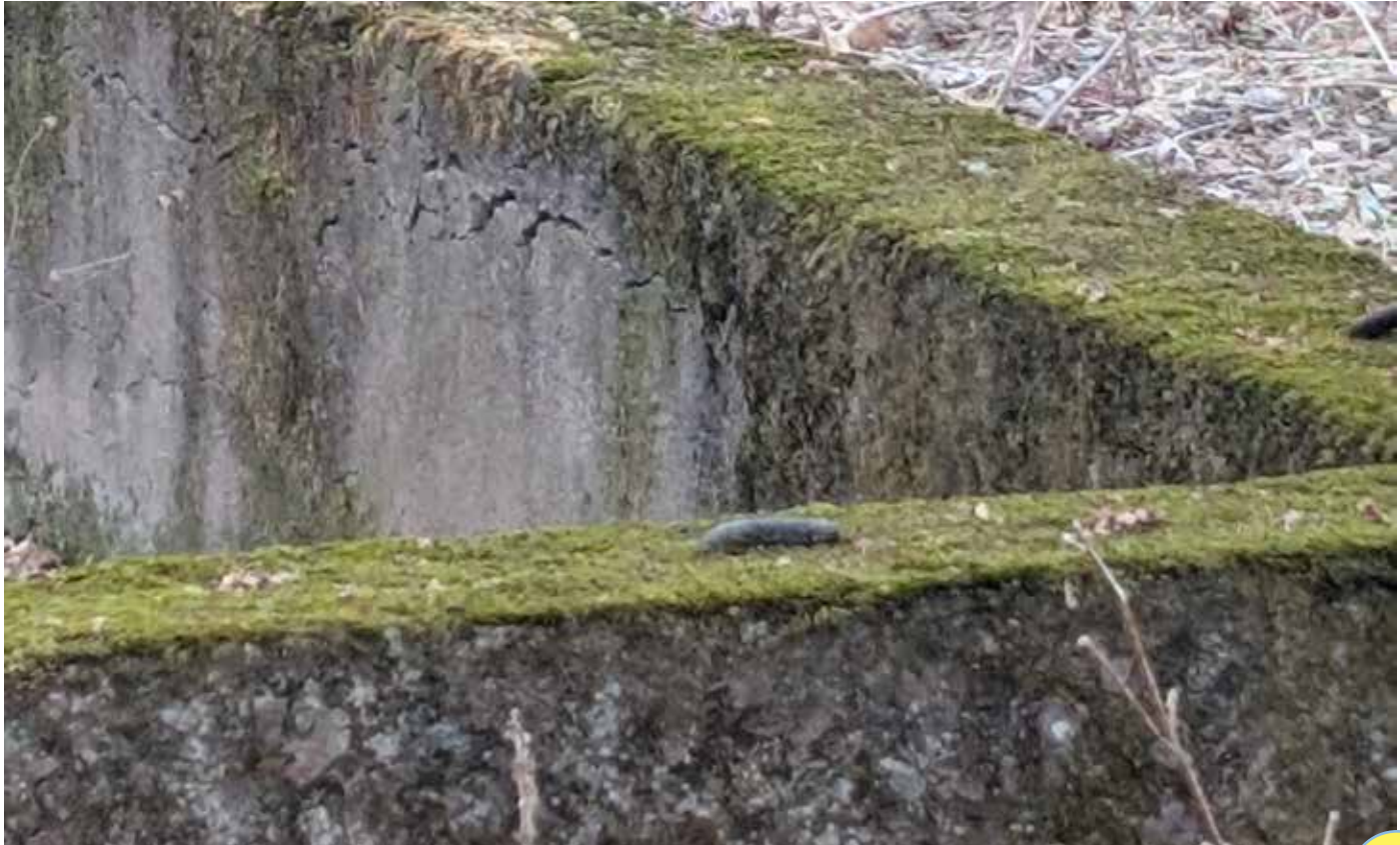
An old concrete wall in the Kirby Park Natural Area
