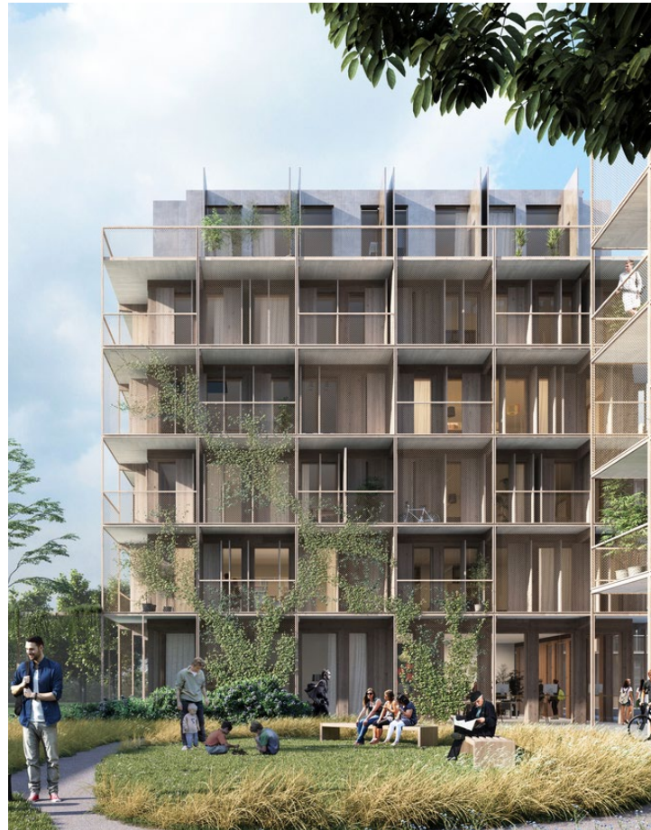
Multifamily, Kjellander Sjöberg Architects
