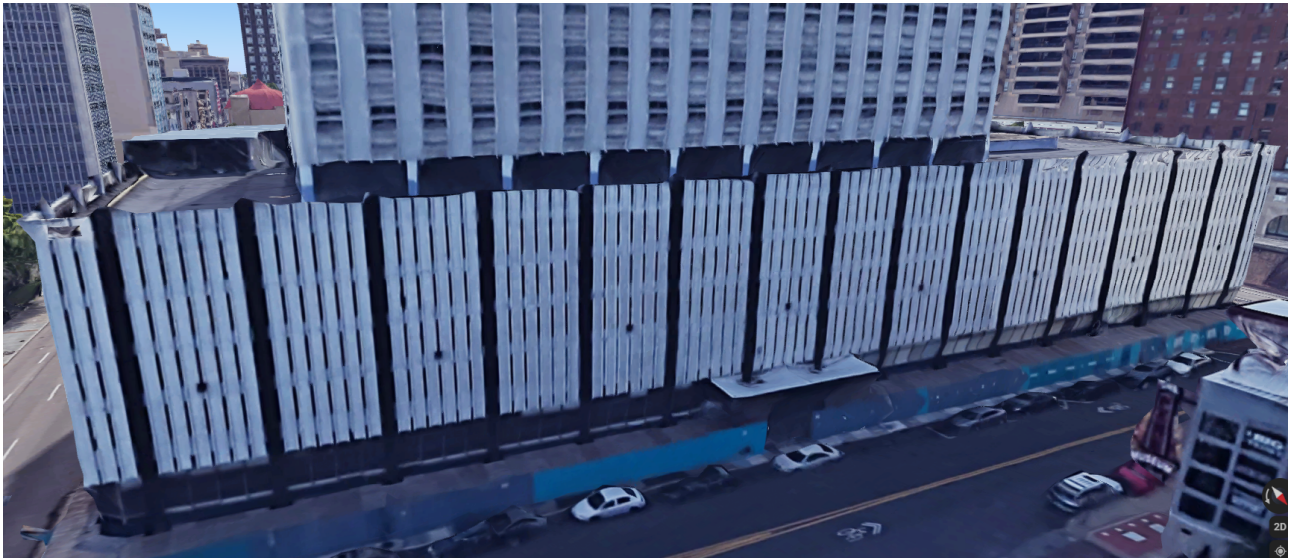
Figure 3: North Elevation – Concrete Podium
