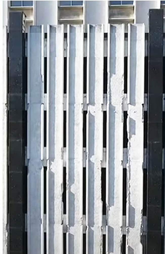
Removal of deteriorating precast concrete elements
