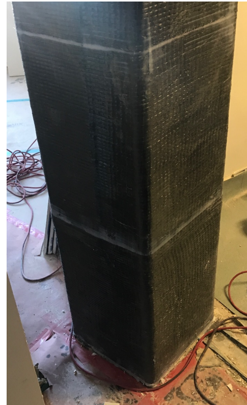
FIBERWRAP APPLICATION ON COLUMN
