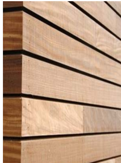
WOOD-1 EXTERIOR TREATED CEDAR RAINSCREEN 2X3 RANDOM LENGTHS MFR: LOCALLY SOURCED STAIN: OLYMPIC NATURAL
