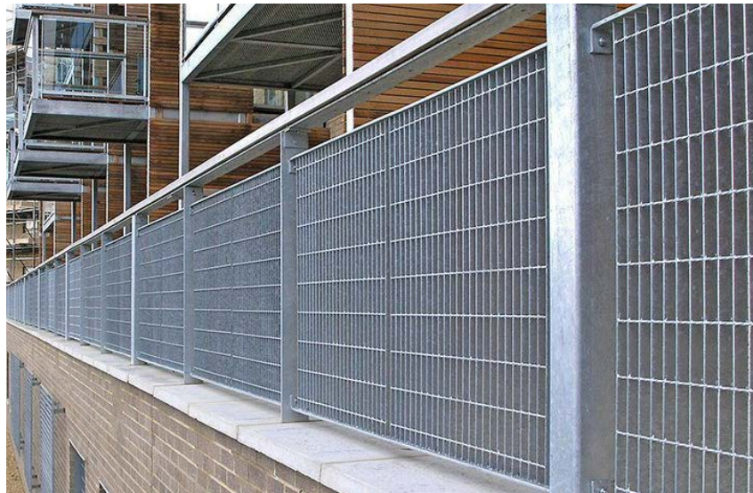
MTL-2 38" HEAVY-DUTY WELDED BAR GRATING APPLIED TO EXISTING GUARDRAIL MFR: MCNICHOLS COLOR: GALVANIZED, POWDER COATED
