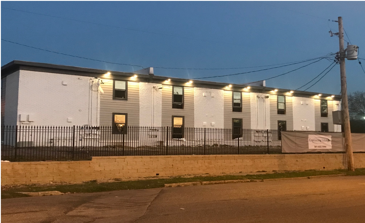
West Elevation South Building off Decatur Street:
