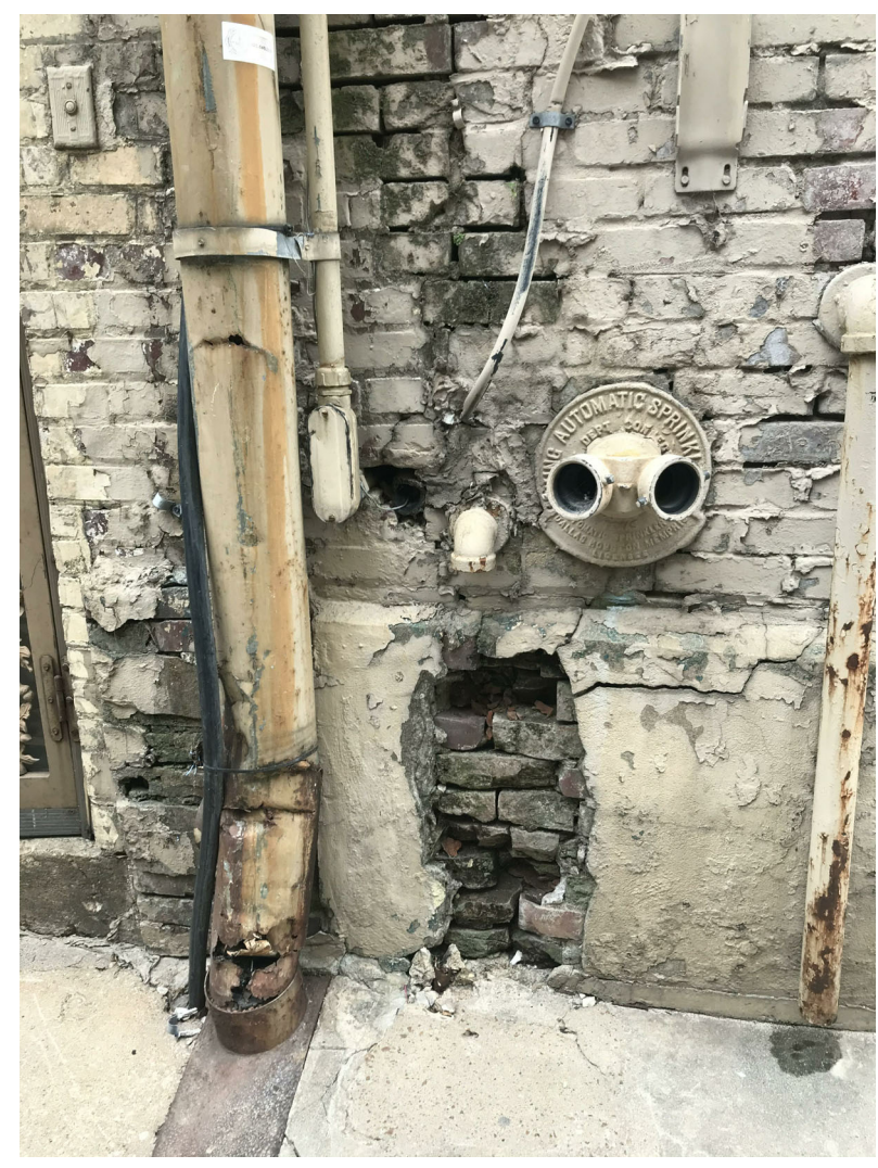
EXISTING FIRE ESCAPE
