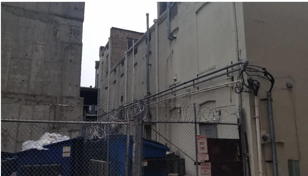
118-124 Monroe Avenue- Rear Façade
