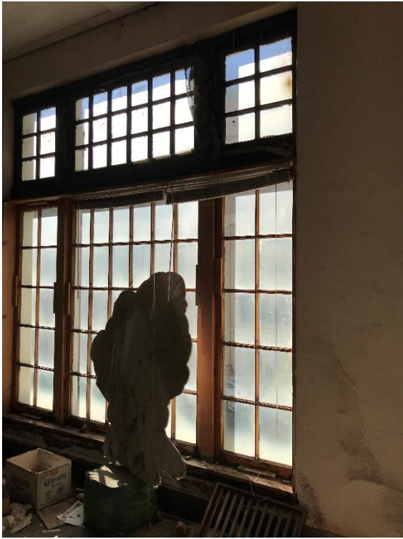
Upper Floor Condition
