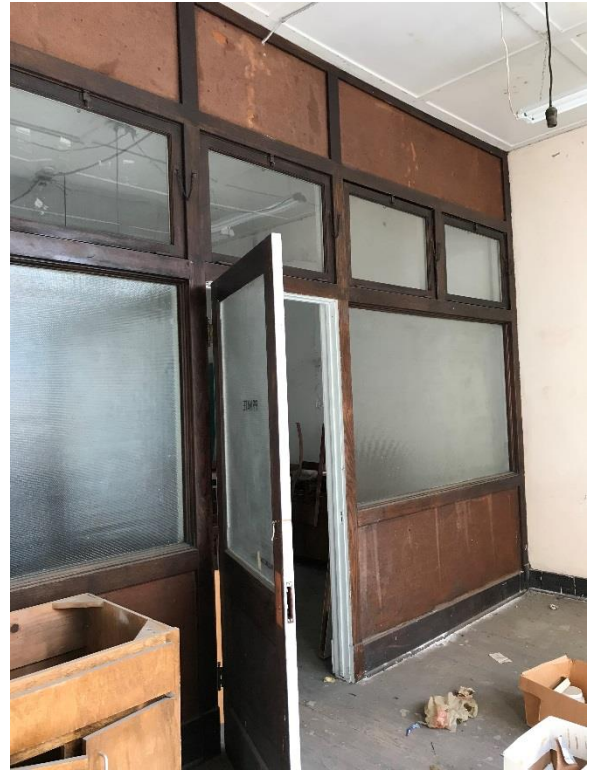
Upper Floor Condition
