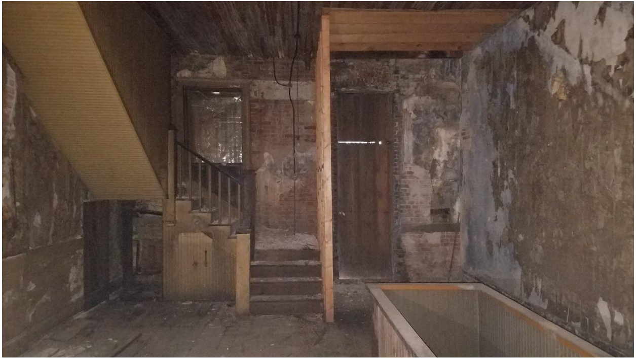
Upper Floor Condition
