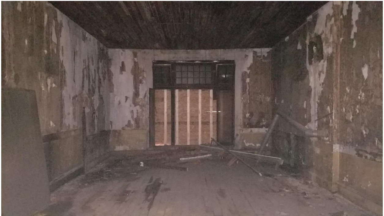
Upper Floor Condition
