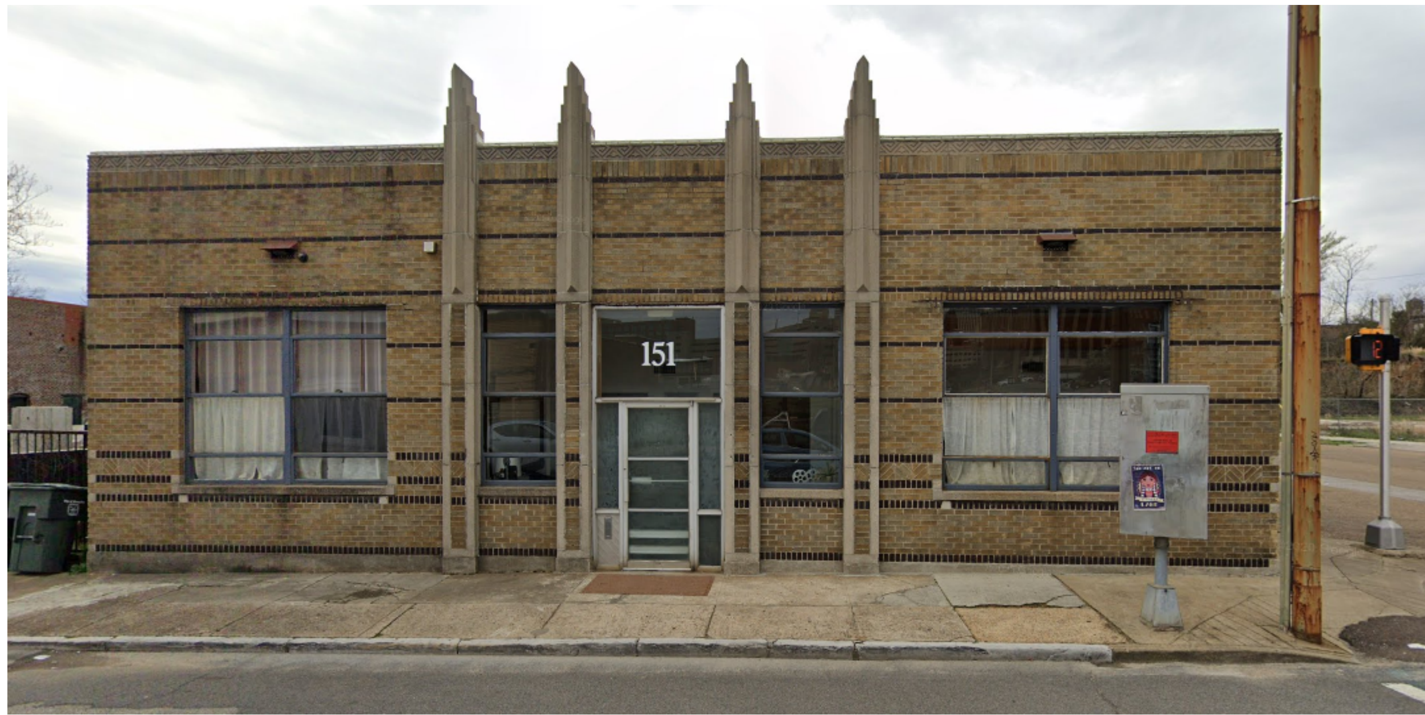
EXTERIOR NORTH ELEVATION
