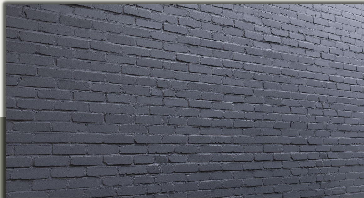
5. Building Exterior: Paint New & Existing Brick & Stone Pilasters
