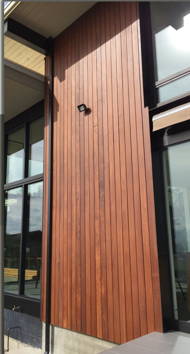
2. Walgreens Storefront: Composite Wood Installation
