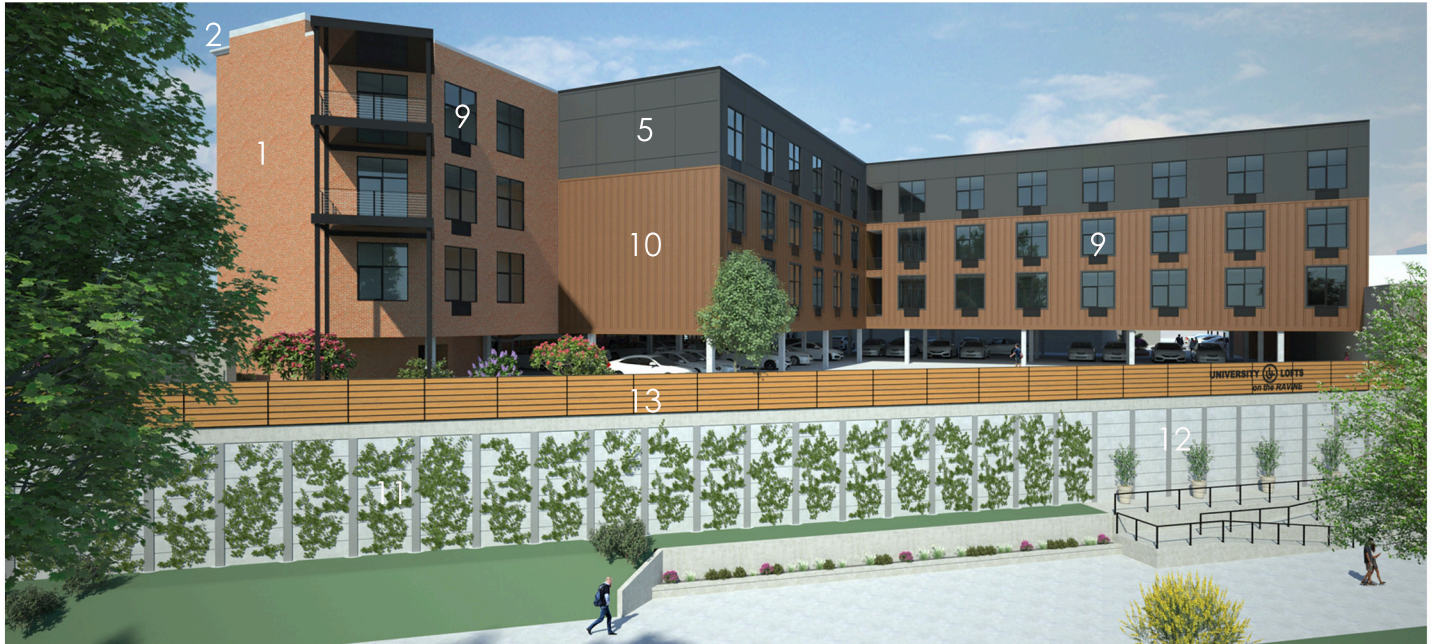
NORTH AND EAST FACADES: FROM THE RAVINE
