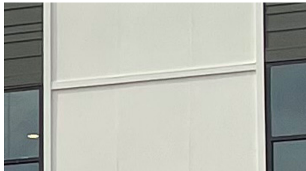
PAINTED PANEL & TRIM
