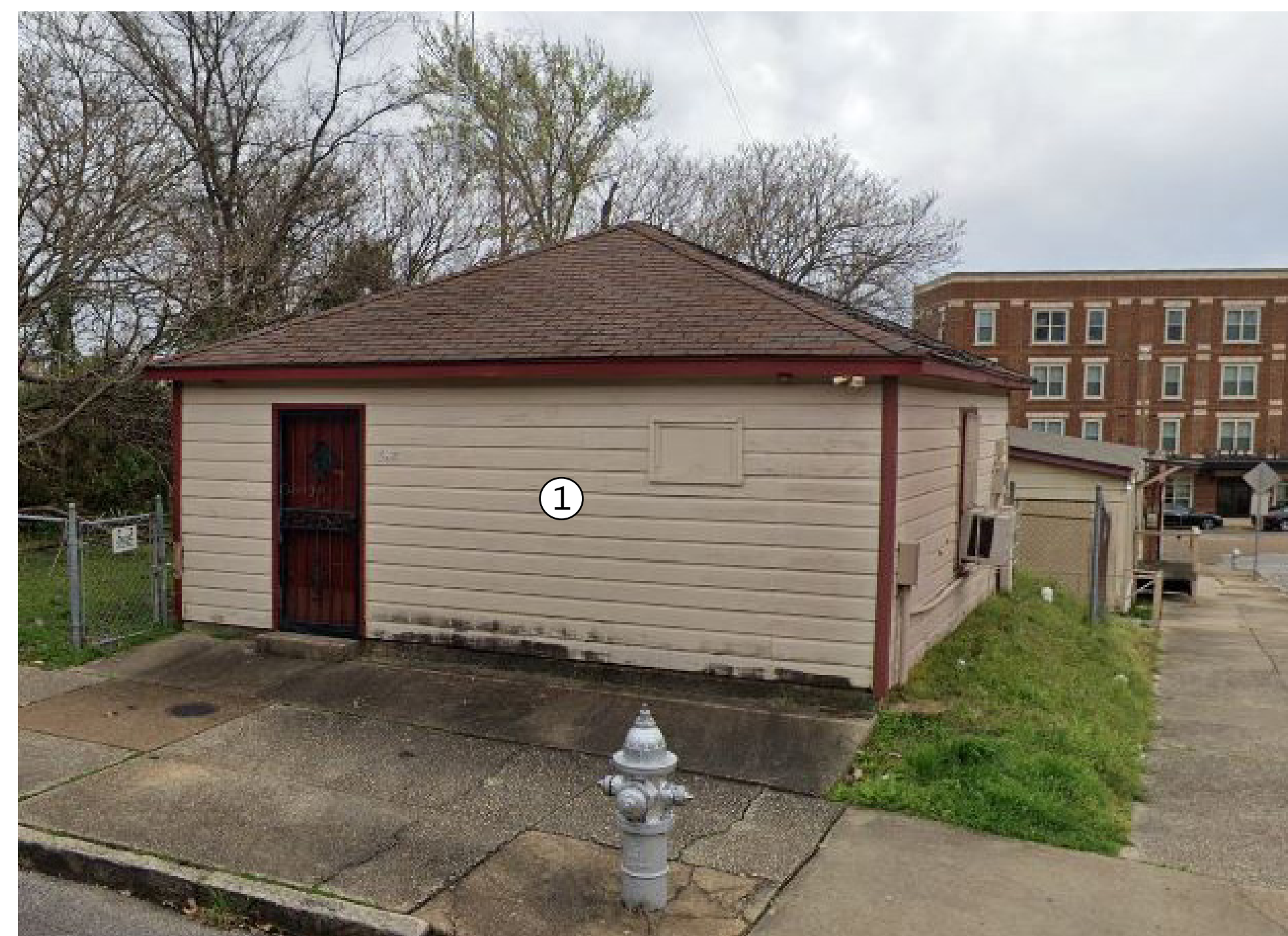
WLOK STORAGE FACILITY
