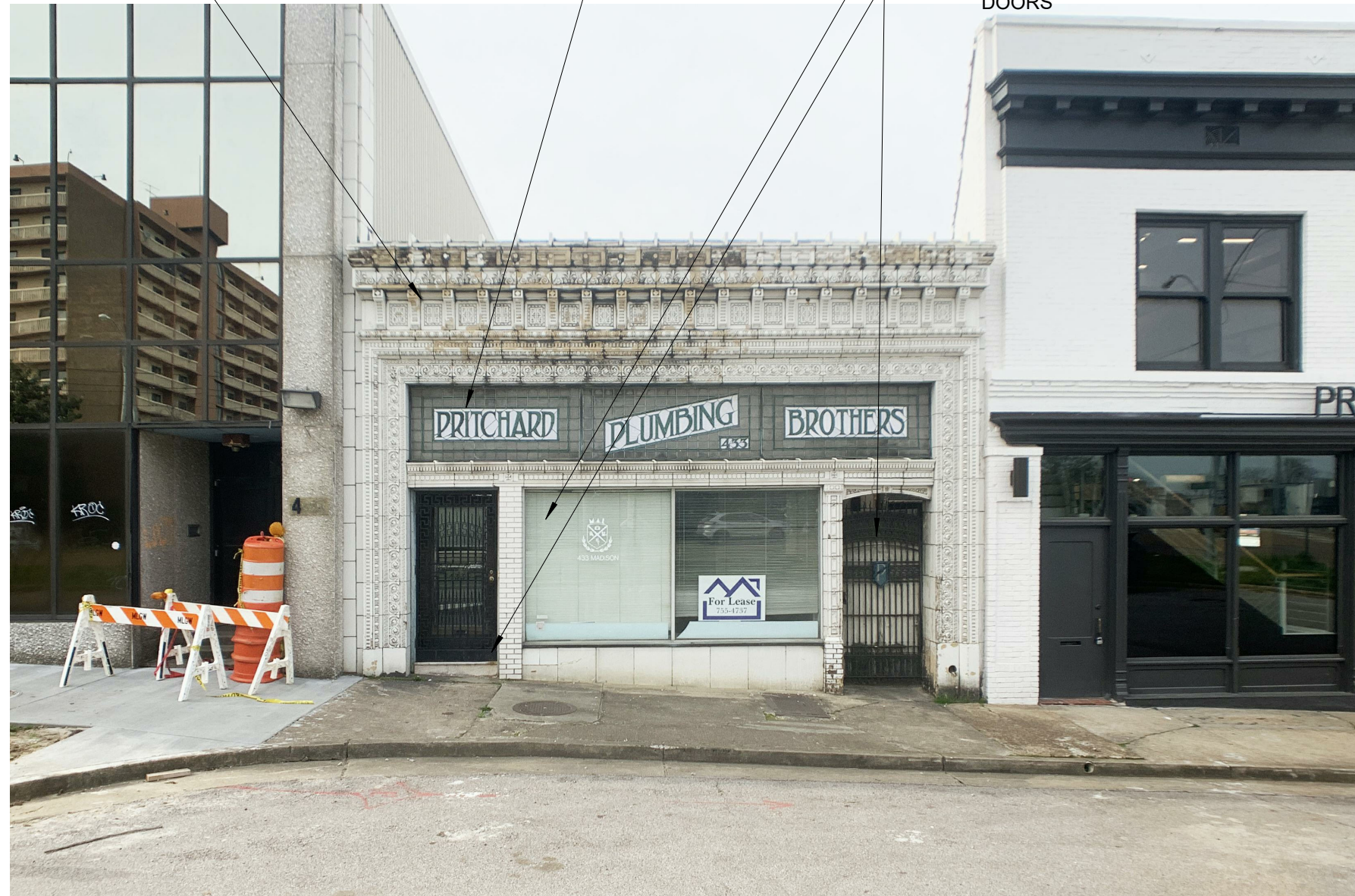
EXISTING GLAZED TERRA-COTTA MASONRY
