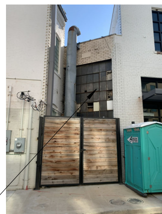
EXISTING SOUTH WINDOW
