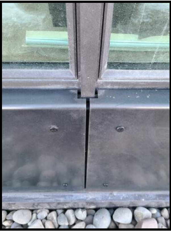
INSTALLATION DETAILS - JOINT
