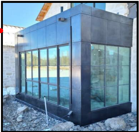
Weathered Black Dark Stainless Cladding with exposed fasteners (see Detail)
