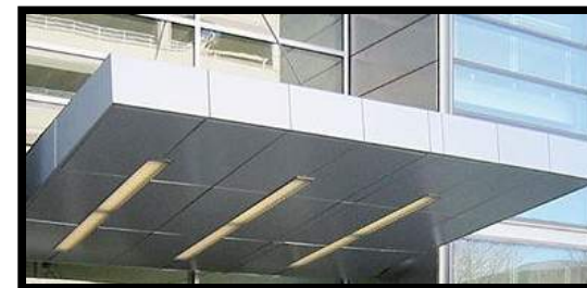
Aluminum Clad Roof Canopy
