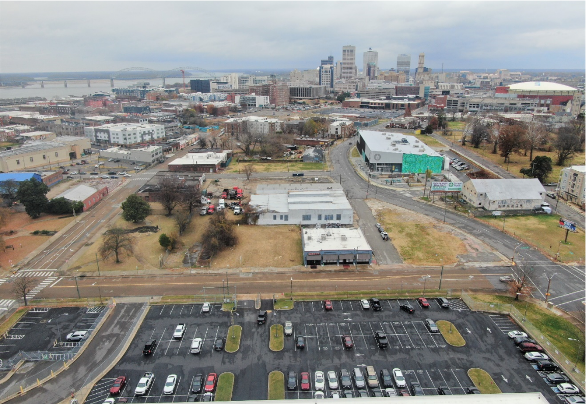
Overall Site Facing North
