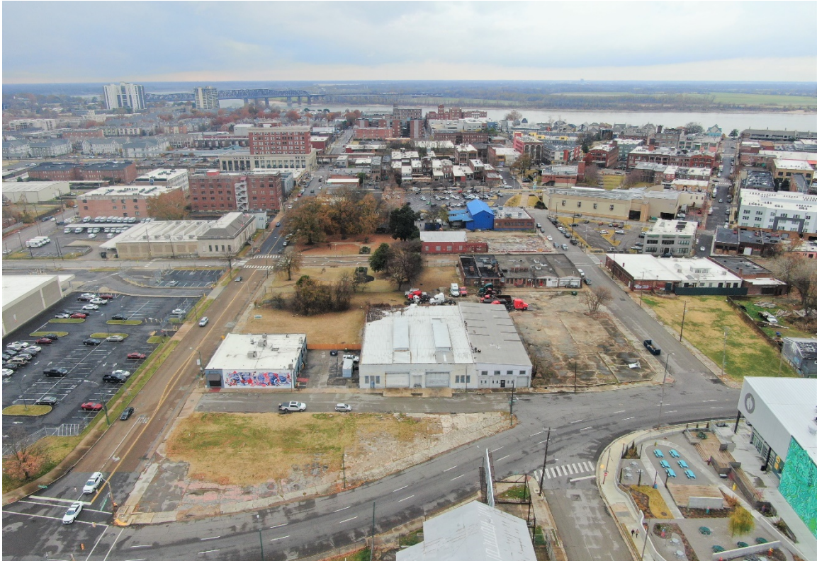
Overall Site Facing West
