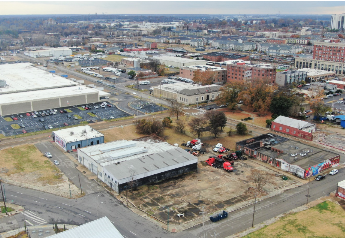
Overall Site Facing Southwest
