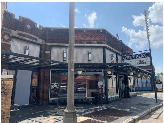
Masonry repairs / tuckpointing will be completed along with structural reinforcement. All masonry joints will be ground minimum of 1"-1 1/4" on substantial majority of facade. Parapet cap, limestone "diamonds," and various decorative limestone architectural features will be repaired or replaced, to match original construction, as feasible.
