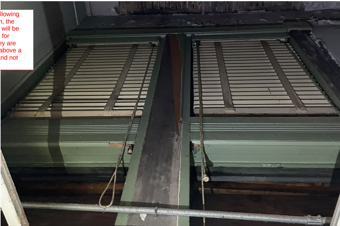
West (Primary) Elevation - Remnant framing of historic windows above ceiling line
