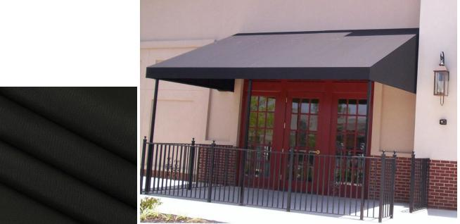
Style of the deep awning at the small eastern patio by Memphis Sweets. 8'8" (I) X 28' (w) bolted to the building facade and the concrete landing. Black sunbrella fabric will be used to recover the existing metal frame awning covered in red fabric. Black sunbrella fabric
