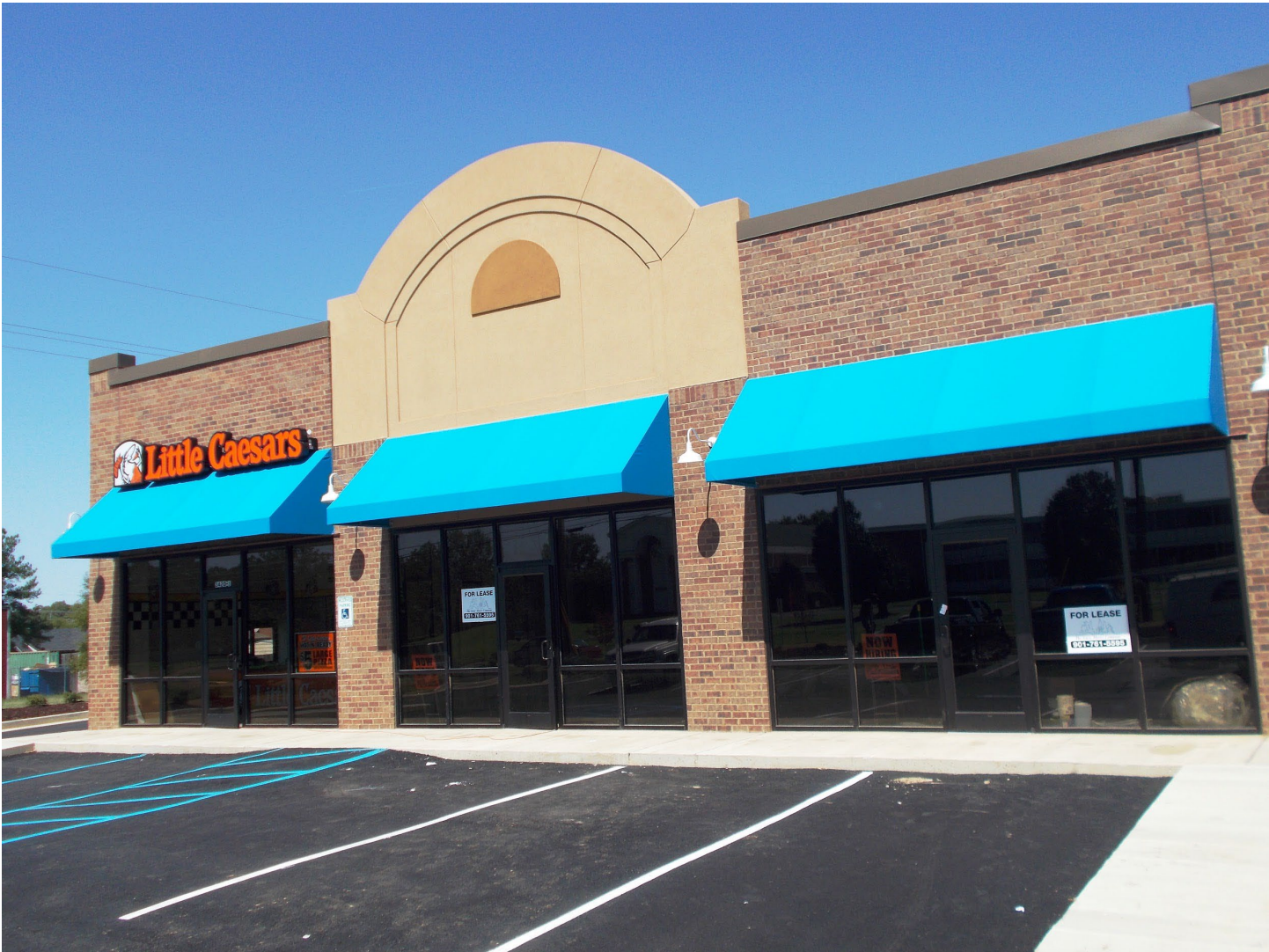
*Black* fabric Awning will replace the red ones.
