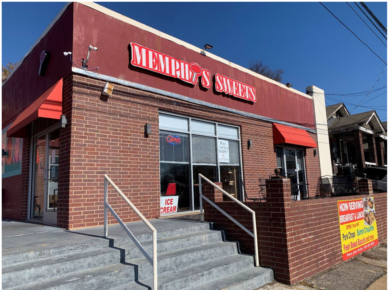
Photographs of existing conditions
