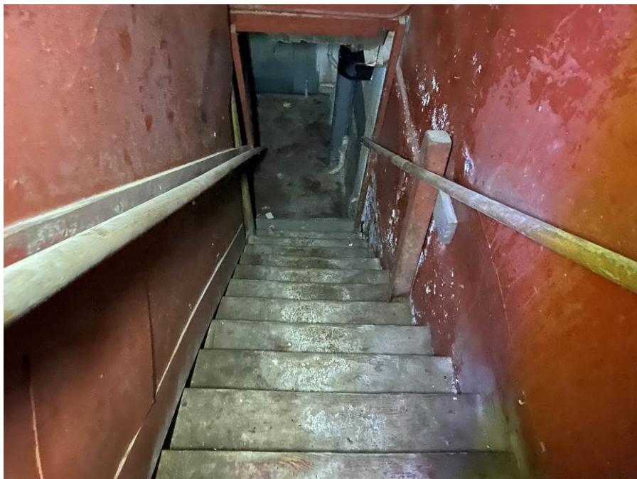
Photo 34 Stair to Basement in 80 North Main
