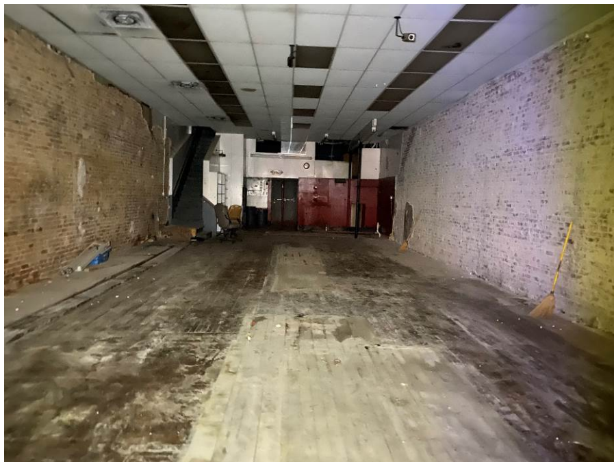
Photo 32 First Floor General Condition of 80 North Main
