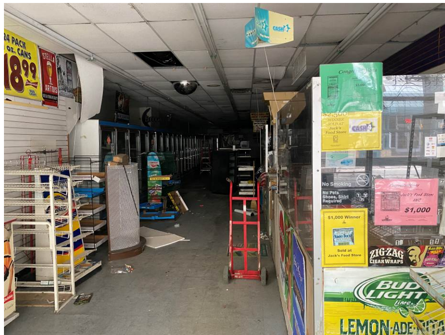
Photo 22 General Condition of 84 North Main Ground Floor
