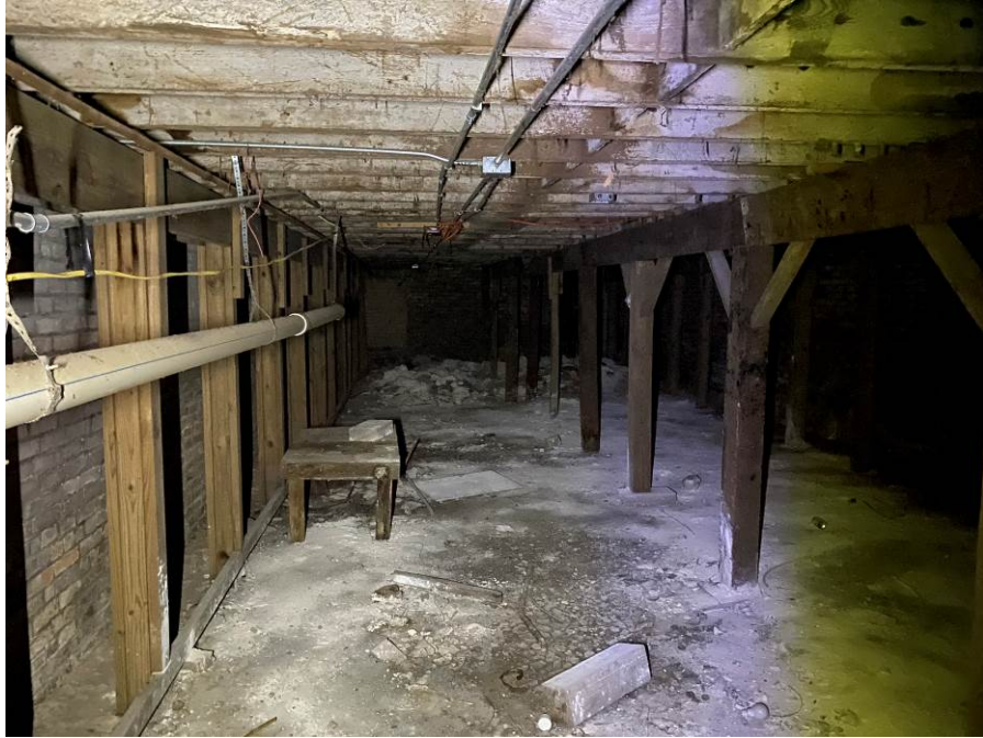
Photo 17 86 North Main Basement Framing
