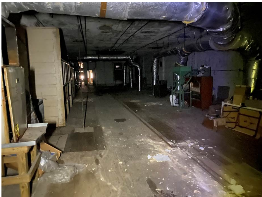
Photo 38 General Condition of 80 North Main Second Floor
