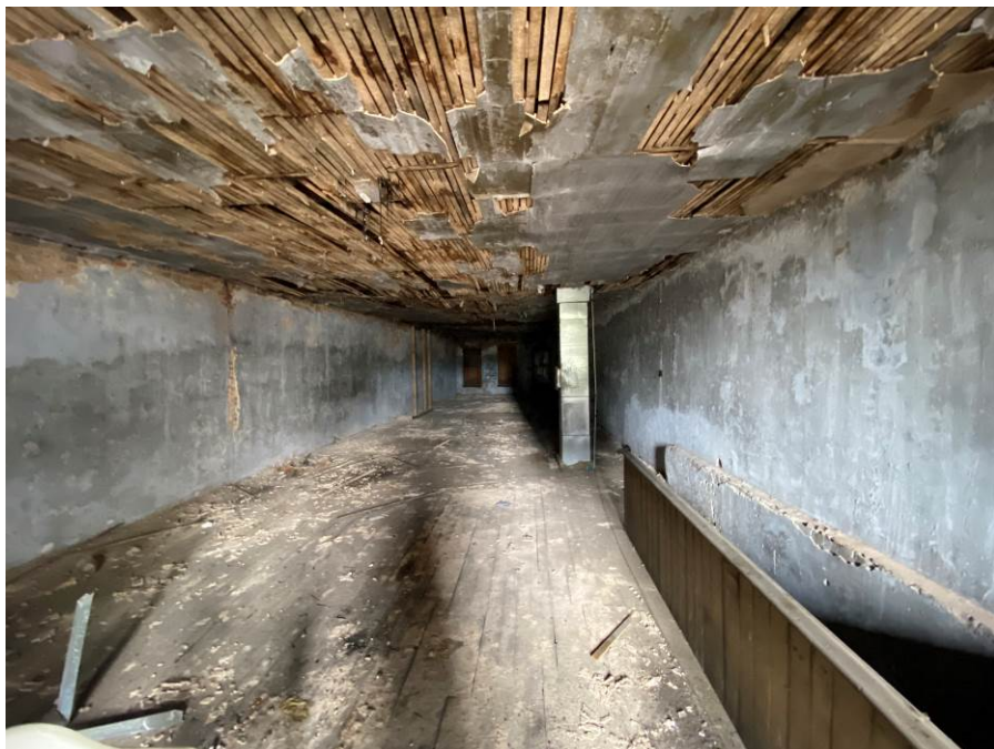
Photo 20 86 North Main General Framing Condition
