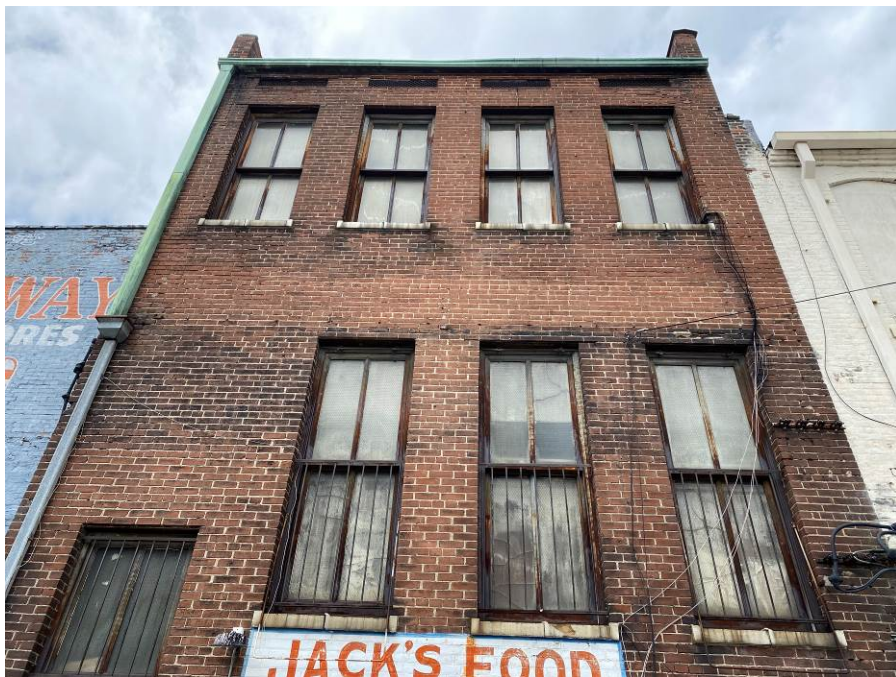
Photo 48 General Condition of Masonry on 84 North Main
