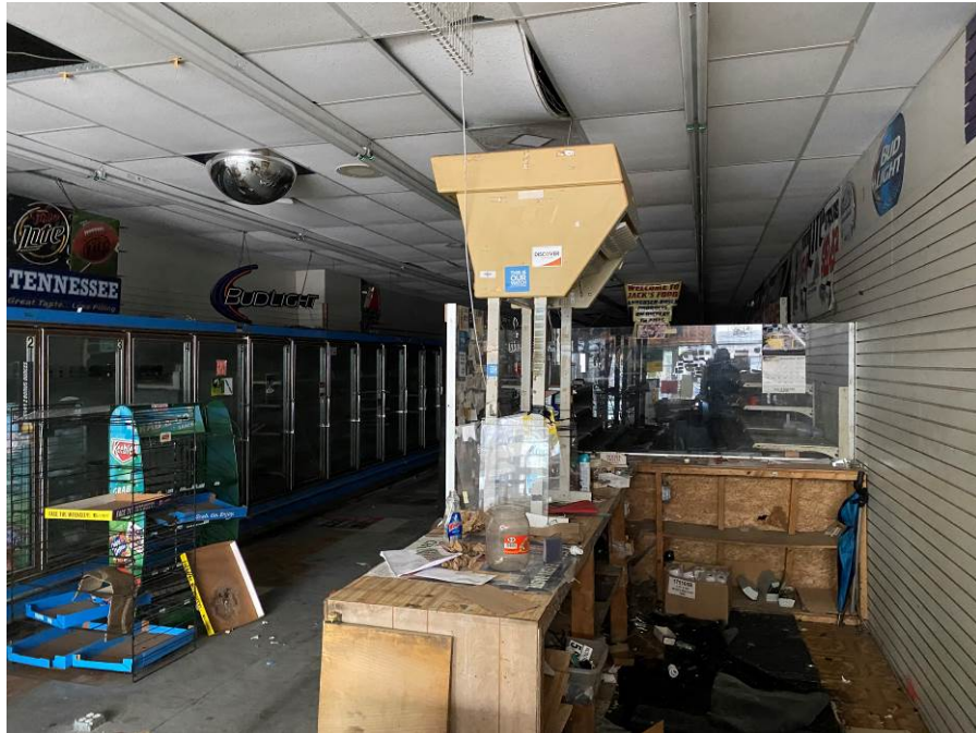
Photo 23 Interior General Condition of Ground Floor at 84 North Main
