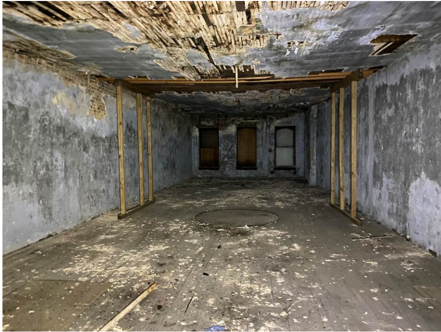
Photo 89 Shoring at Roof of 86 North Main
