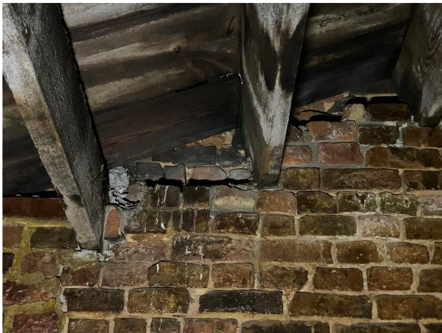
Photo 70 Rotating Joists at Sloped Area on 88 North Main
