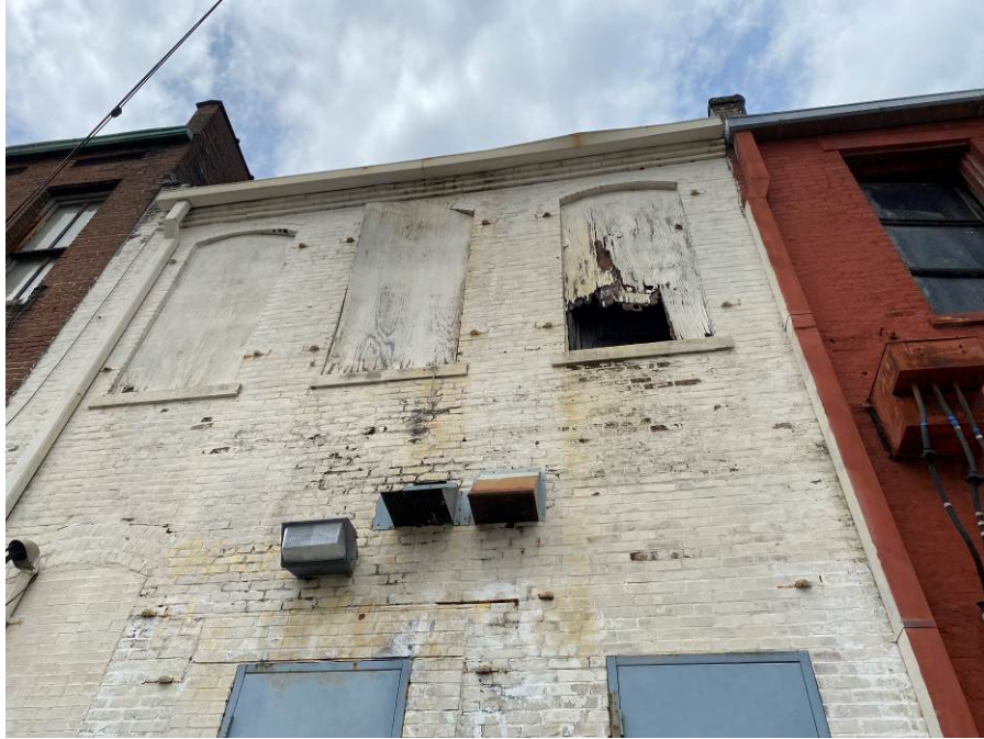
Photo 47 General Condition of Exterior Masonry on Rear of 86 North Main
