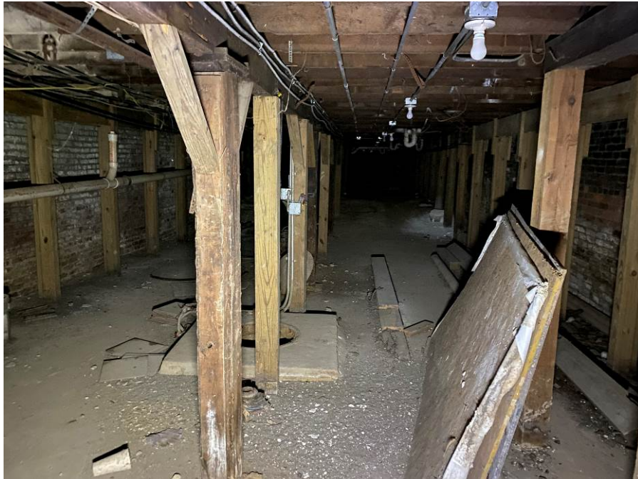
Photo 15 General Basement Condition of 86 North Main
