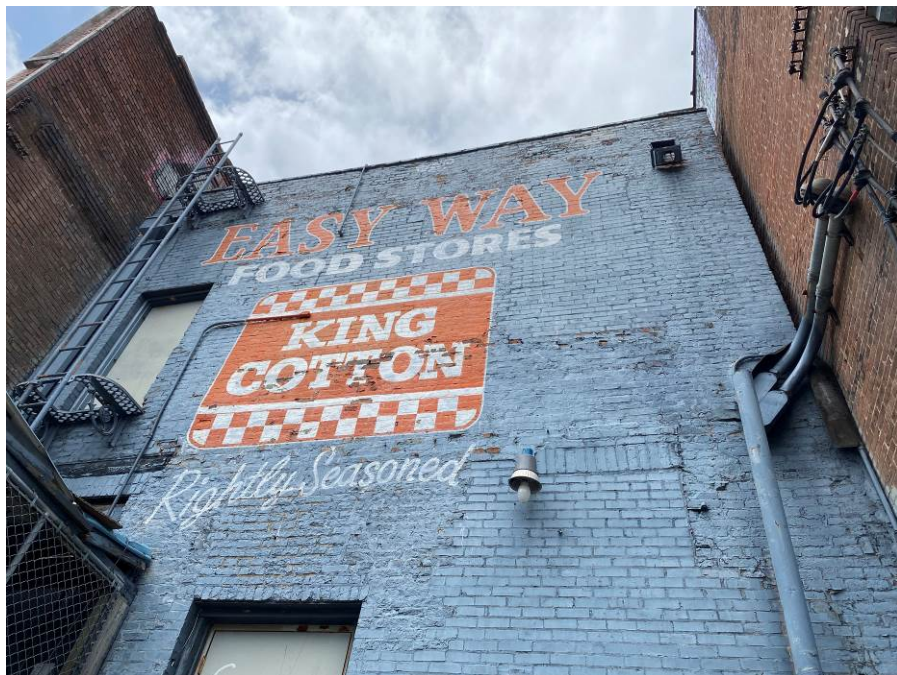
Photo 6 Condition of Masonry at Rear on 80 North Main
