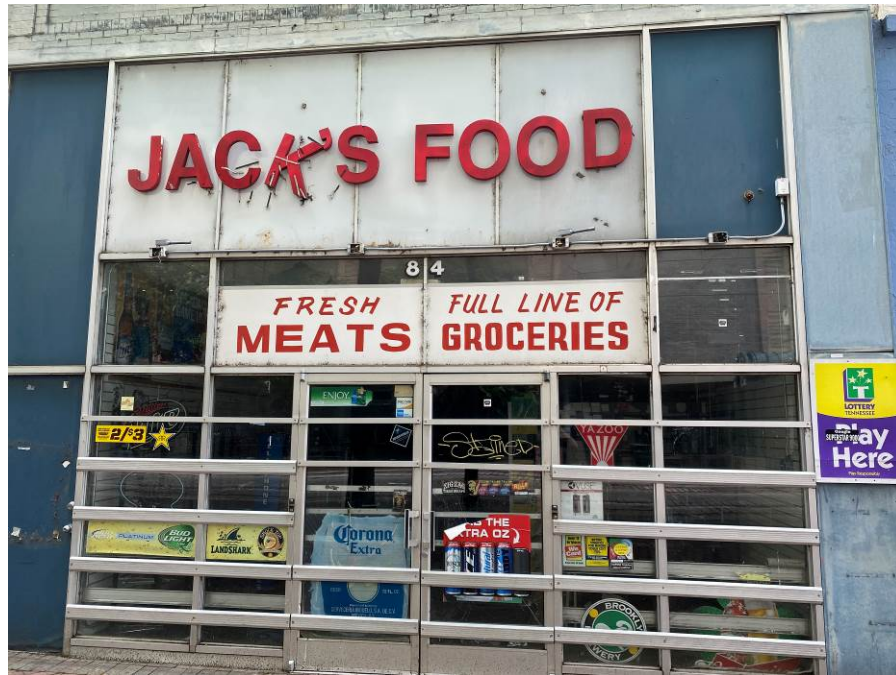
Photo 21 Front Elevation of 84 North Main
