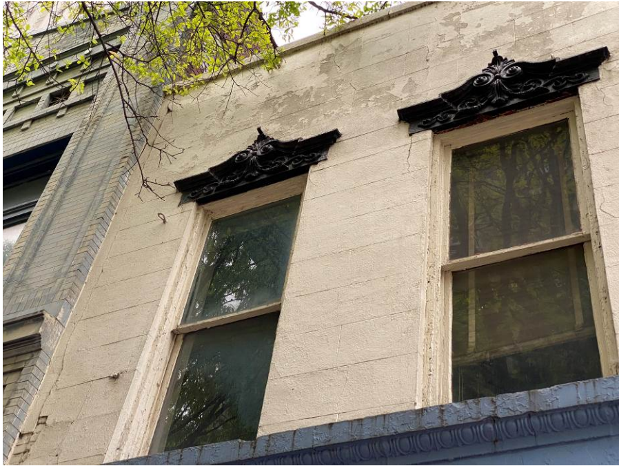
Photo 113 Parging Coat of Masonry Coat on Condition o
