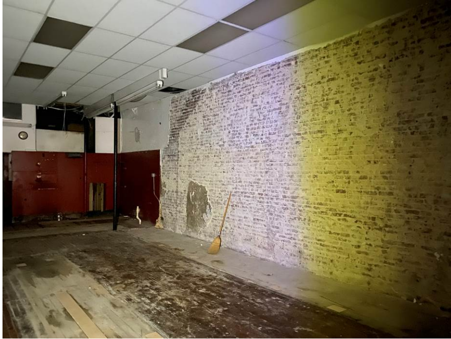
Photo 33 General interior Condition of 80 North Main
