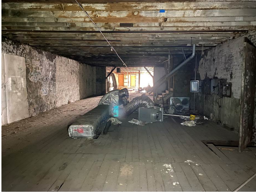
Photo 9 Condition of 88 North Main Second Floor
