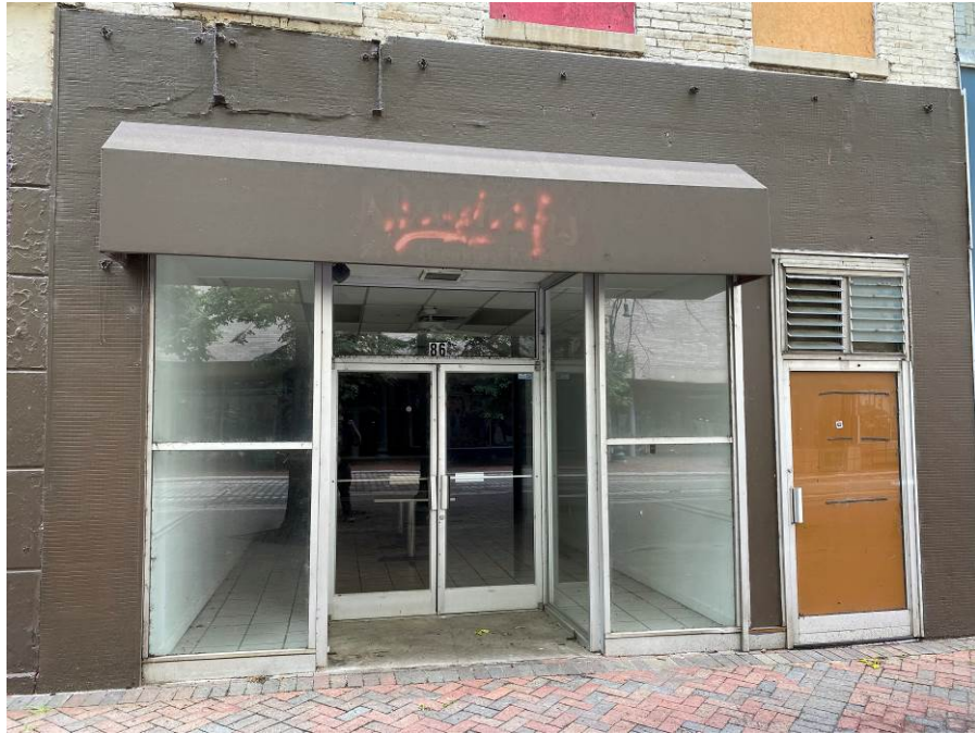
Photo 11 Front Elevation at 86 North Main
