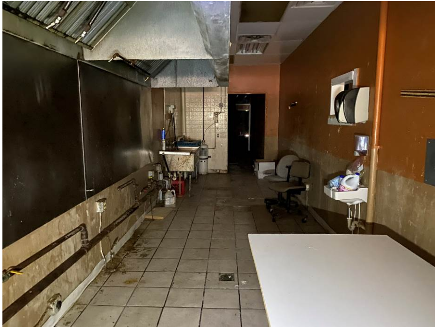
Photo 13 General Interior Kitchen at First Floor of 86 North Main
