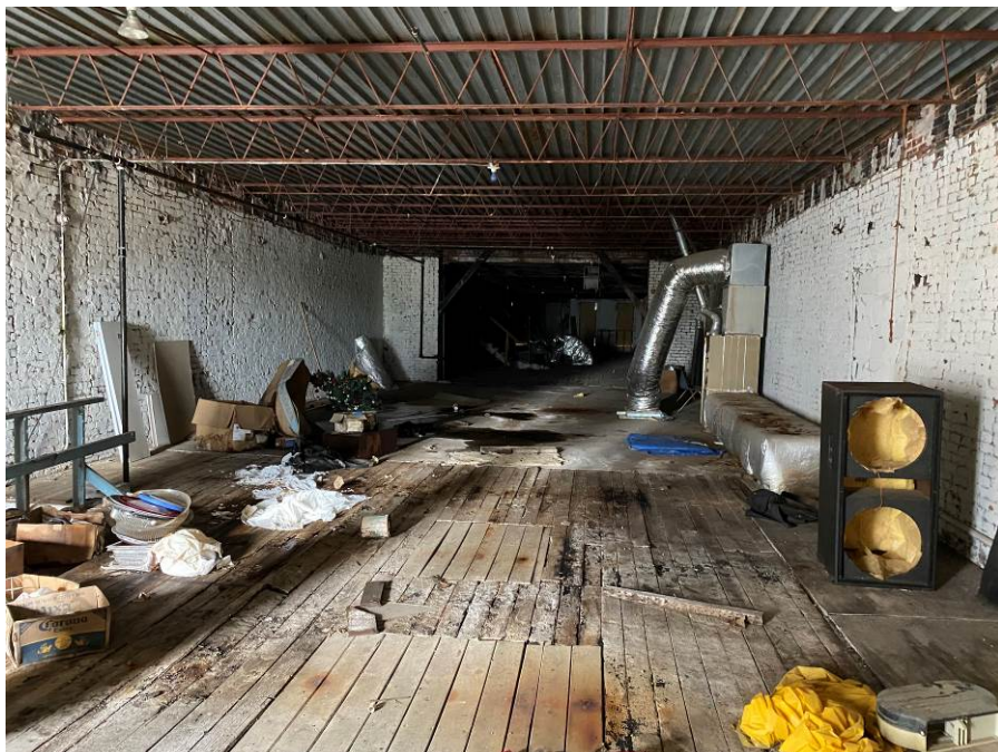
Photo 8 General Condition of 88 North Main Second Floor
