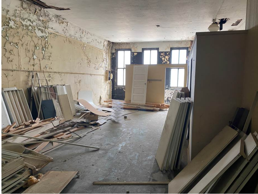
Photo 29 Second Floor Framing at 84 North Main
