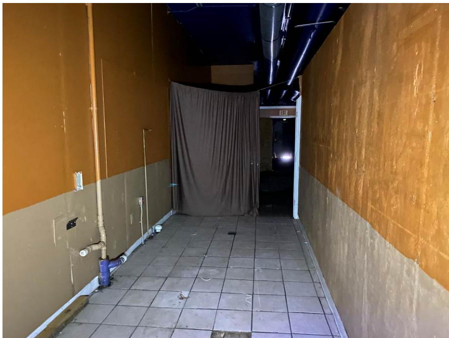
Photo 14 General Condition of 86 North Main
