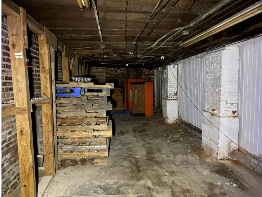
Photo 37 General Condition of Framing in Basement of 80 North Main
