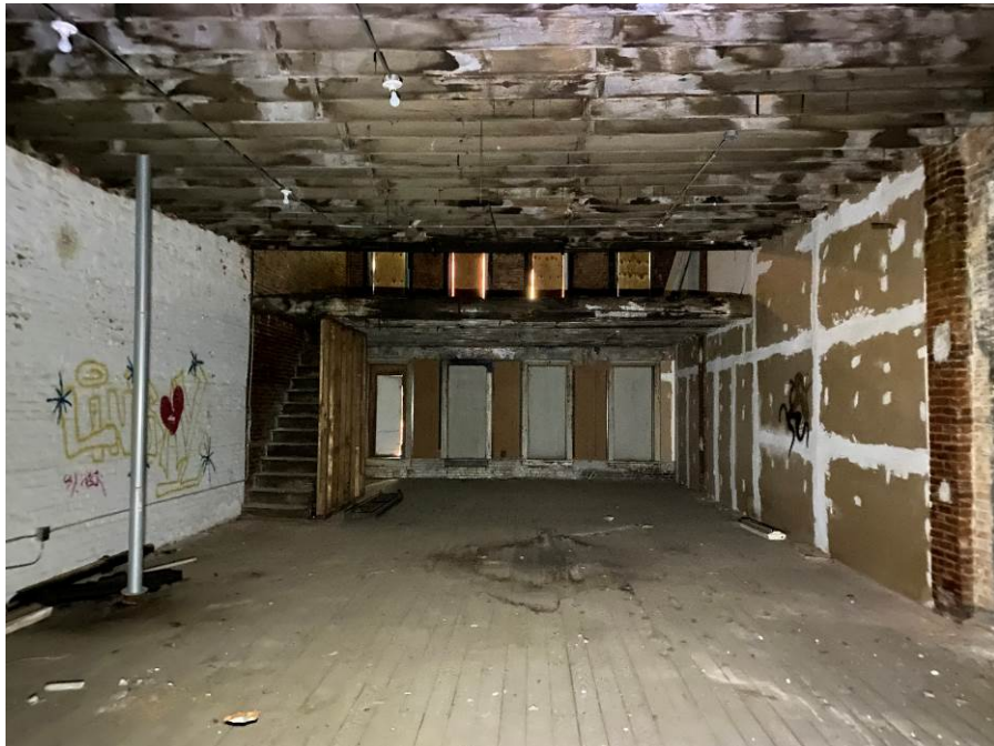
Photo 10 Condition of 88 North Main
