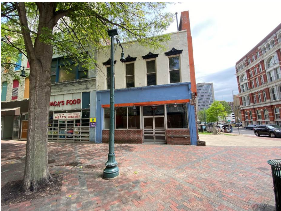
Photo 112 Masonry of 80 North Main
