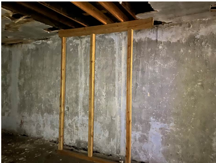
Photo 98 Condition of Temporary Shoring at 86 North Main
