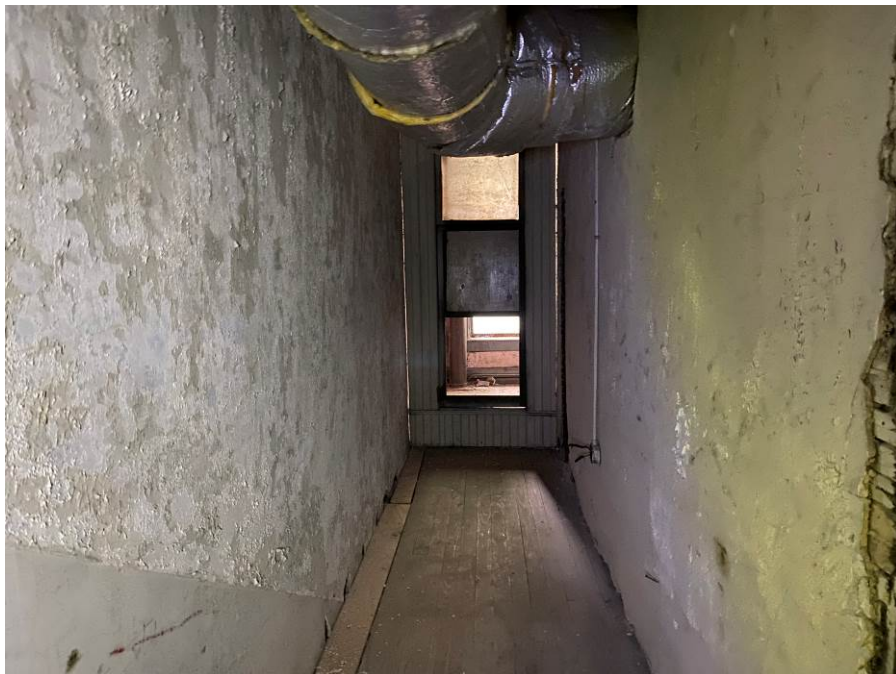
Photo 40 Hallway on Second Floor of 80 North Main
