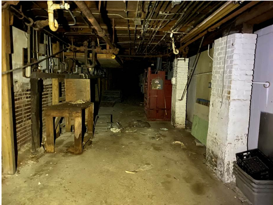
Photo 35 Basement Framing of 80 North Main
