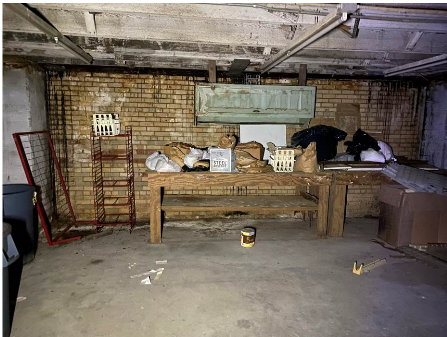
Photo 28 Basement Wall and Framing in 84 North Main
