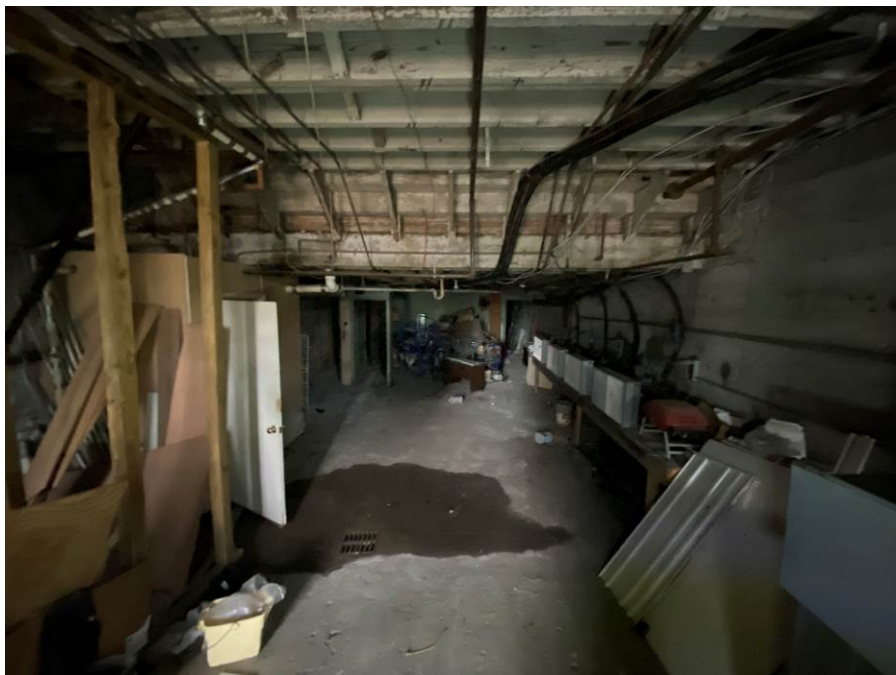
Photo 26 Basement Framing of 84 North Main
