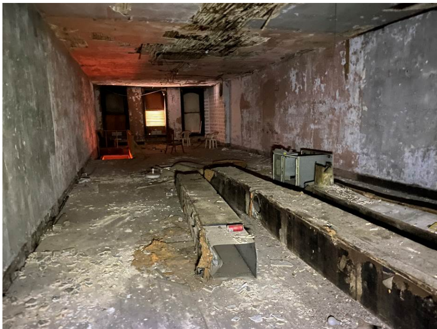
Photo 18 Second Floor Framing General Condition of 86 North Main
