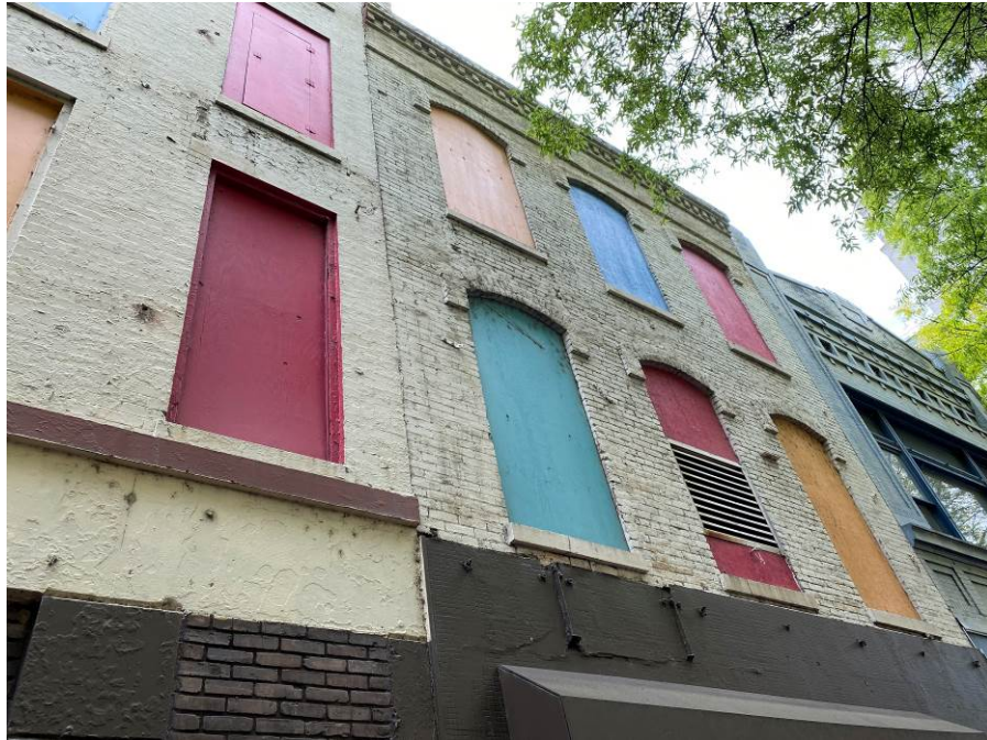
Photo 51 Condition of Masonry
