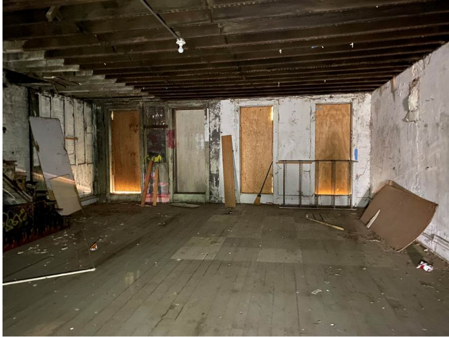
Photo 57 Condition of Window Openings
