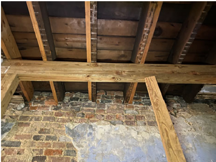
Photo 100 Shoring Bearing Condition at 86 North Main
