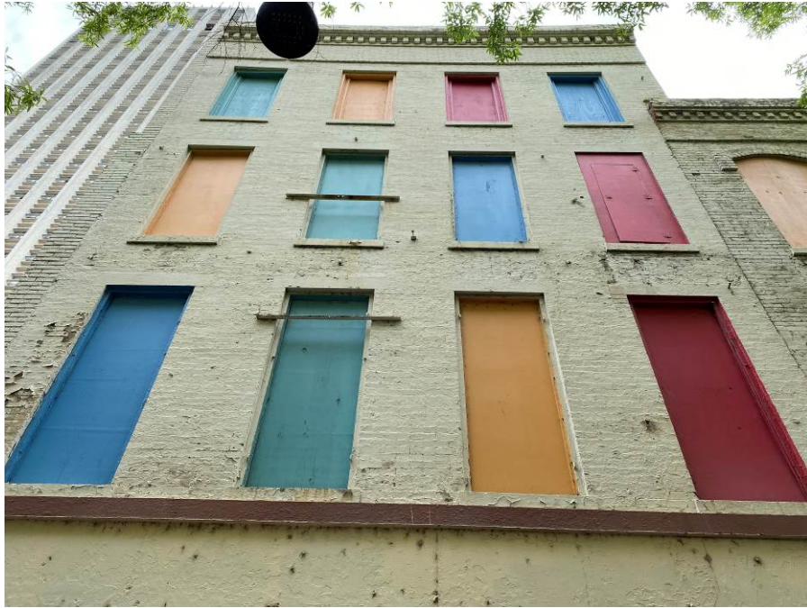
Photo 49 Masonry Condition on 88 North Main Elevation
