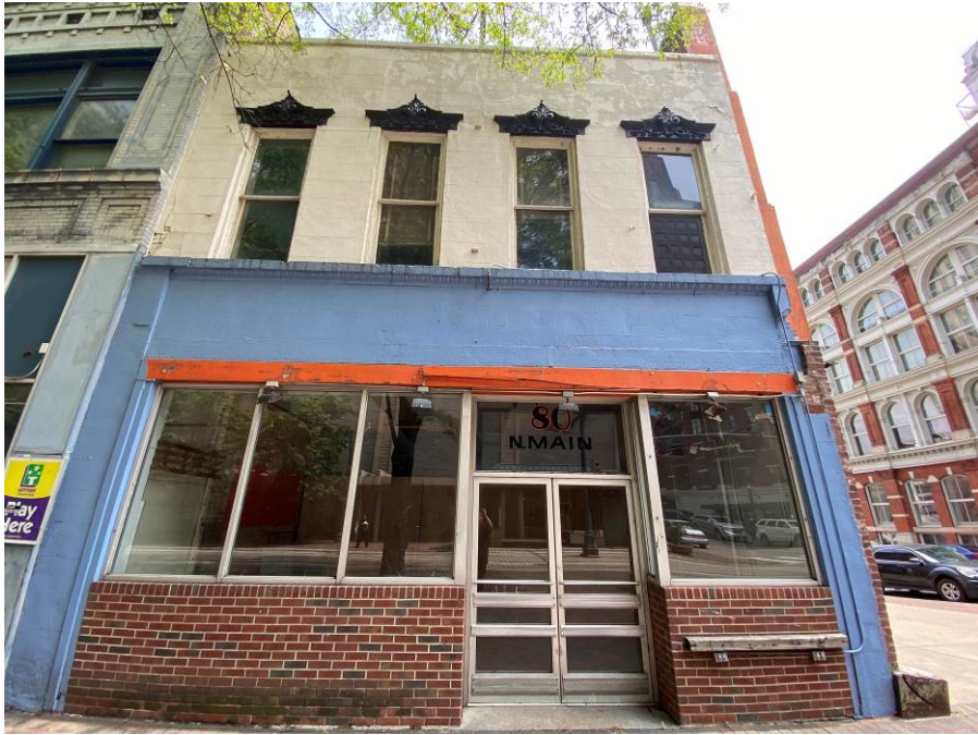
Photo 111 Exterior Condition of 80 North Main
