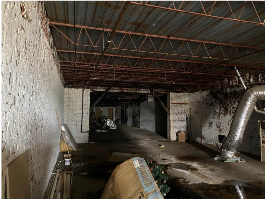
Photo 53 Condition of Second Floor Addition Framing on 88 North Main
