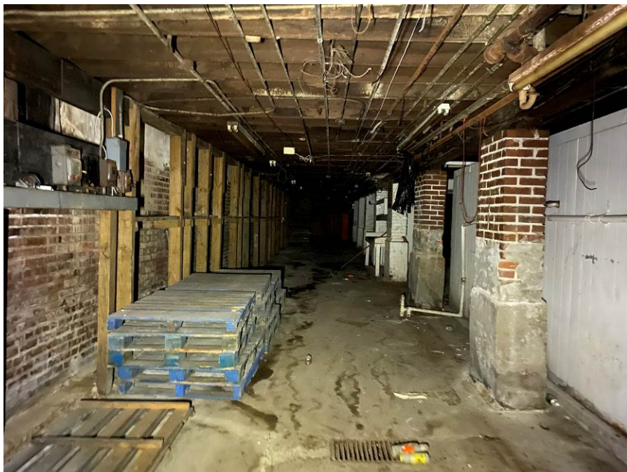
Photo 36 Masonry Pilasters in Basement of 80 North Main
