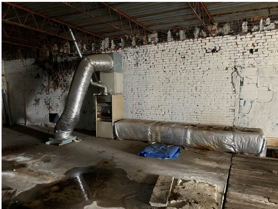
Photo 54 Metal Deck and Steel Bar Joists on 88 North Main
