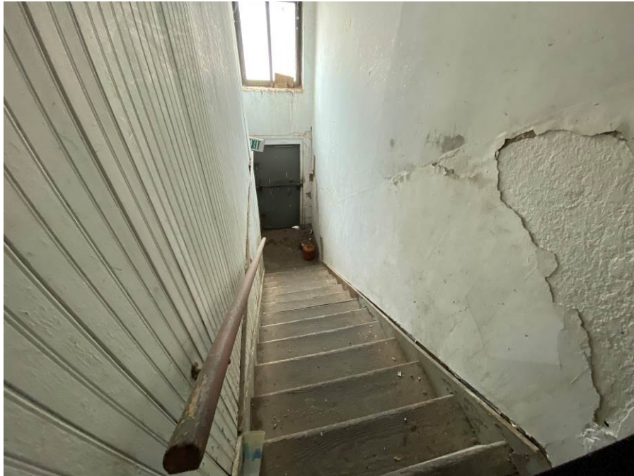
Photo 25 Stairwell at 84 North Main Rear
