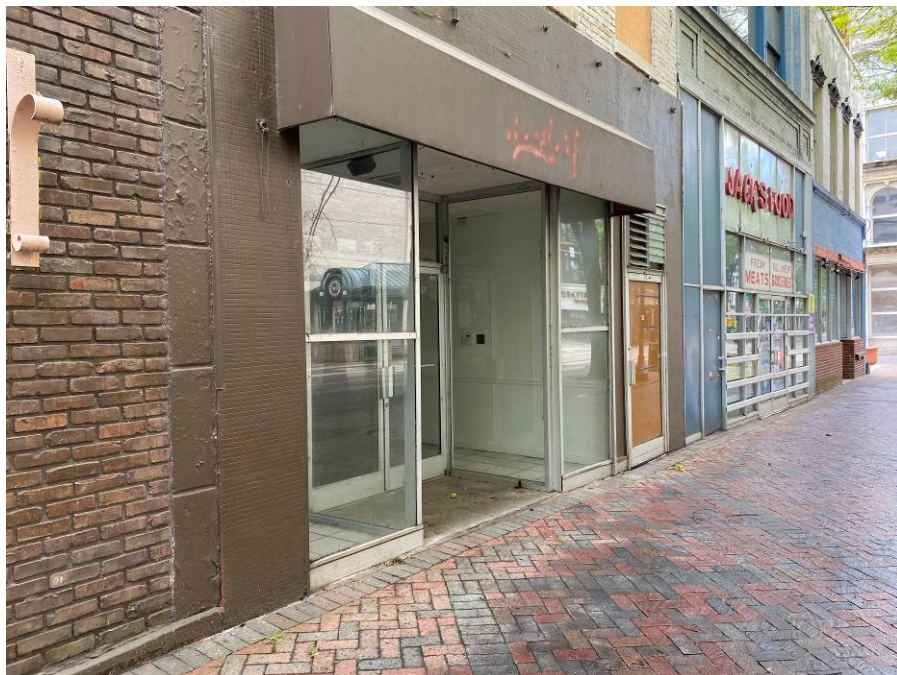
Photo 4 Front Elevation of 86 North Main
