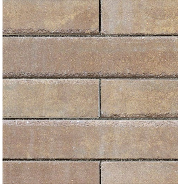
Entry and Courtyard Paving: Custom Brick, 3.5" x 20"
