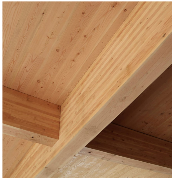
Exposed Structure: Mass Timber, S. Yellow Pine
