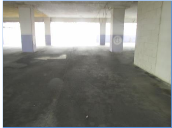
Pavement conditions at level 8 of the parking garage
