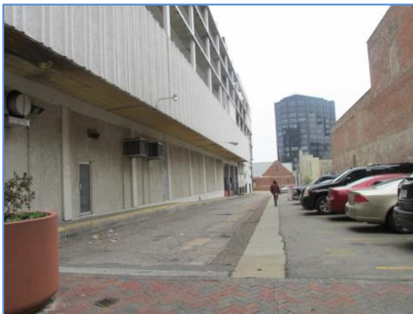
Alley on the south side of the building, facing east and sloping to the south/southeast
