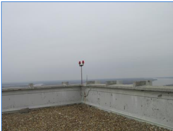
Close up view of the roof surface, parapet and concrete coping
