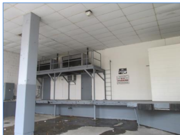
The loading dock on the south side of the building
