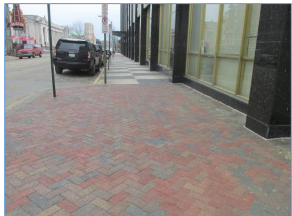
Brick and black and white aggregate sidewalk, north side of the building, looking east
