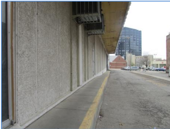
Concrete sidewalk along alley on the south side of the building, looking east
