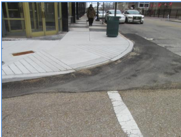
Accessible curb ramp at the public sidewalk on the northeast corner of the site
