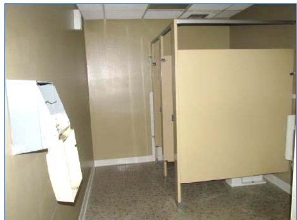
Common area restroom finishes on an upper floor
