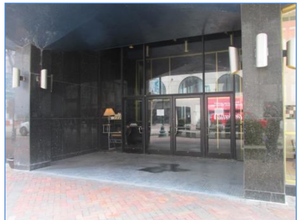
Building-mounted lighting fixtures at pedestrian entrance along Main Street
