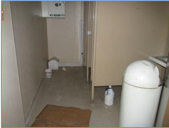
Common bathroom finishes in the lower lobby level
