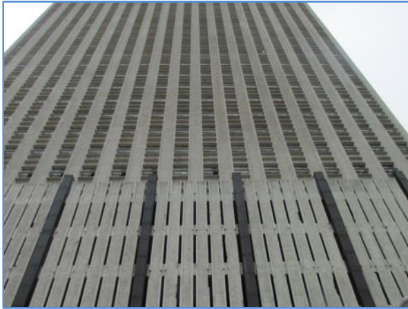
The concrete façade on the north side of the building; note marble panels on the lower level
