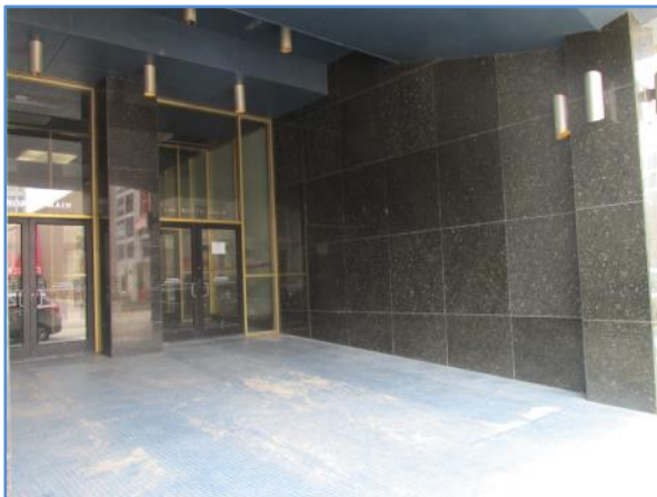
Building-mounted lighting fixtures at pedestrian entrance along Adams Avenue
