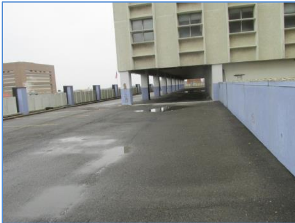
Exposed surface at level 8 of the parking garage
