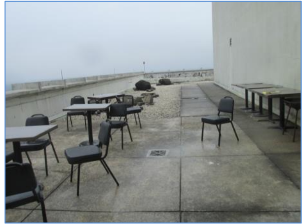
Another view of the concrete pavers and outdoor seating area for the rooftop lounge
