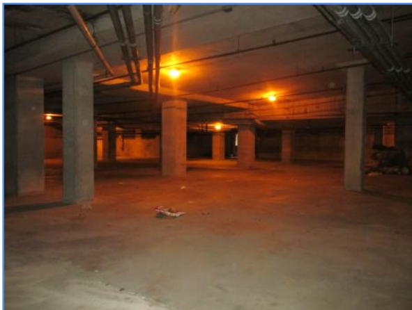
Another view in the lower level of the parking garage/basement
