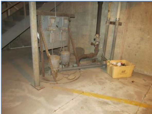
Basement sump area in the parking garage
