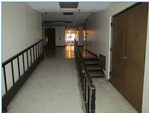
Common corridor at the lower lobby entrance at the parking garage
