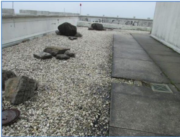
View of the flat, built up roof surface with concrete pavers
