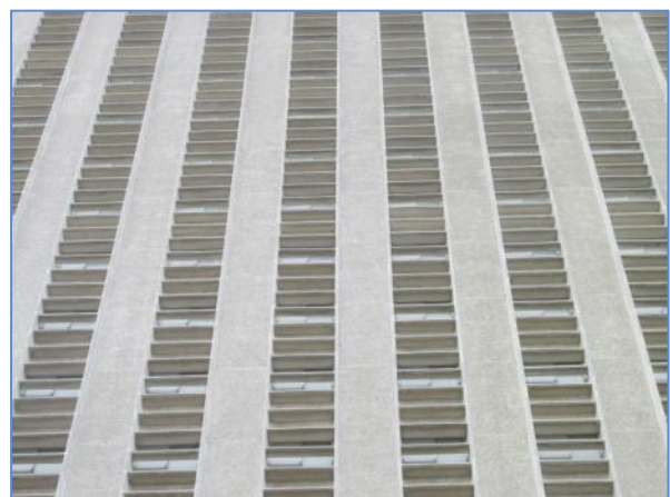
Close up view of the upper level facades on the north side of the building
