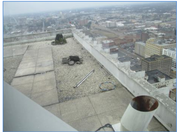
Another view of the roof surface with concrete pavers
