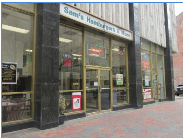
Storefront windows and doors at restaurant on southwest corner of building
