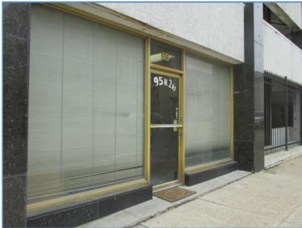
Storefront type windows and doors at southeast corner of building
