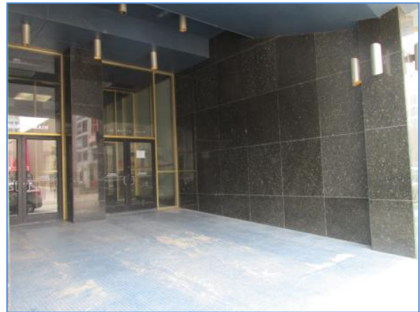
Main pedestrian entrance finishes on the north side of the building
