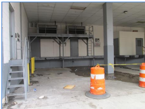
Loading dock on south side of building
