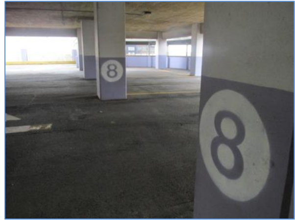
View at level 8 of parking garage
