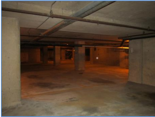
View at basement level of parking garage
