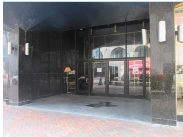
Flush-mounted pedestrian entrance on the west side of the building
