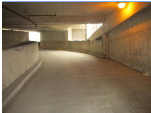
Concrete ramp accessing lower lobby level of parking garage
