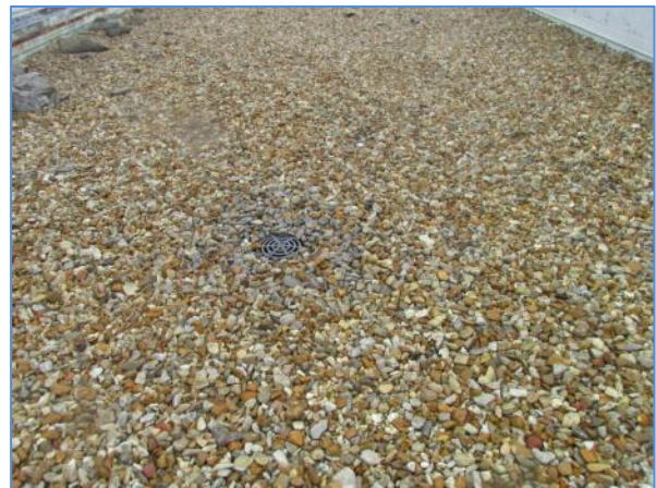
Close up view of the roof surface and internal roof drain
