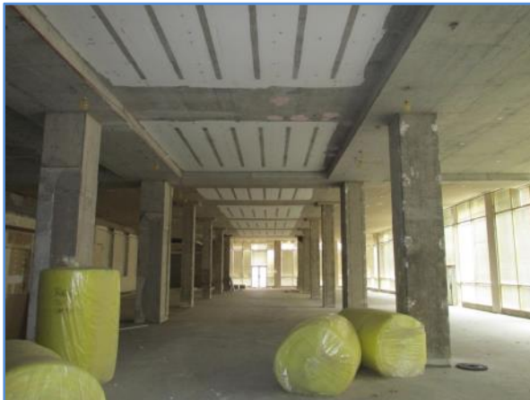
Vacant tenant space on the ground floor
