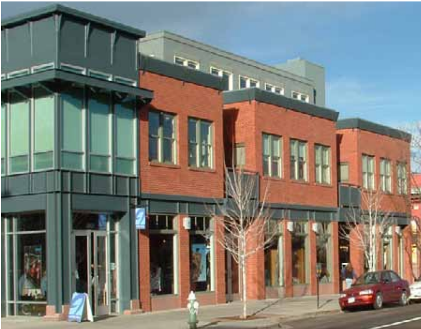
Design floor to floor heights to establish a sense of scale and reflect Memphis traditions.
