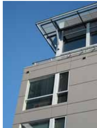
Finished concrete, with scoring details is appropriate.
