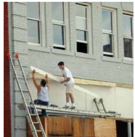
Replace a character-defining feature accurately.
