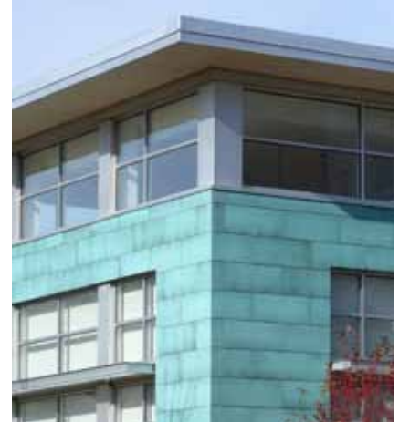
The material should maintain an intended finish over time or acquire a patina. This copper cladding is an example.
