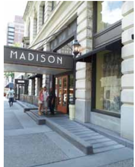
Accessibility improvements should minimally impact the historic character of the building.
