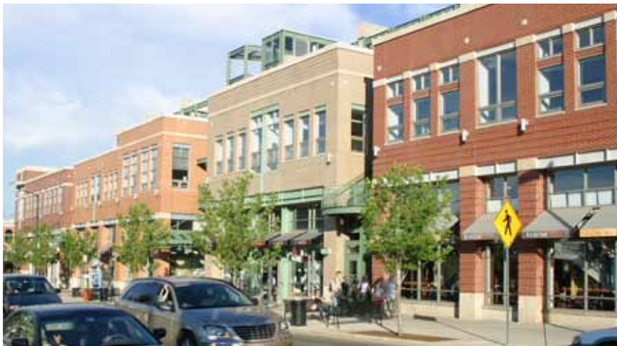
The massing of a parking structure should appear similar in scale to other active use buildings in the area. (This structure has an interior parking deck behind the “wrap” of articulated storefronts, while the exterior reflects facade widths that are typical of the area.)
