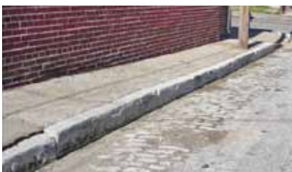
Historic streetscape features such as granite curbs and cornerstones should be preserved.
