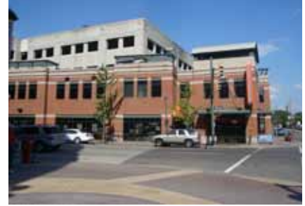
Parking garages screened with buildings or ground floor uses help to maintain the scale of an urban street.
