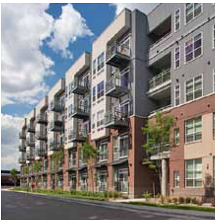
These examples illustrate new buildings that respect the key features of their contexts.
