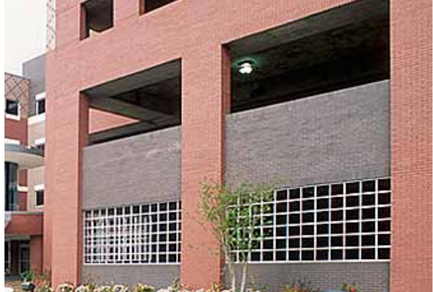
On a secondary street, other methods of providing visual interest may be employed. In these locations, use architectural details. It should include decorative patterns, railings and details to provide visual interest. (This screen design is an example.)
