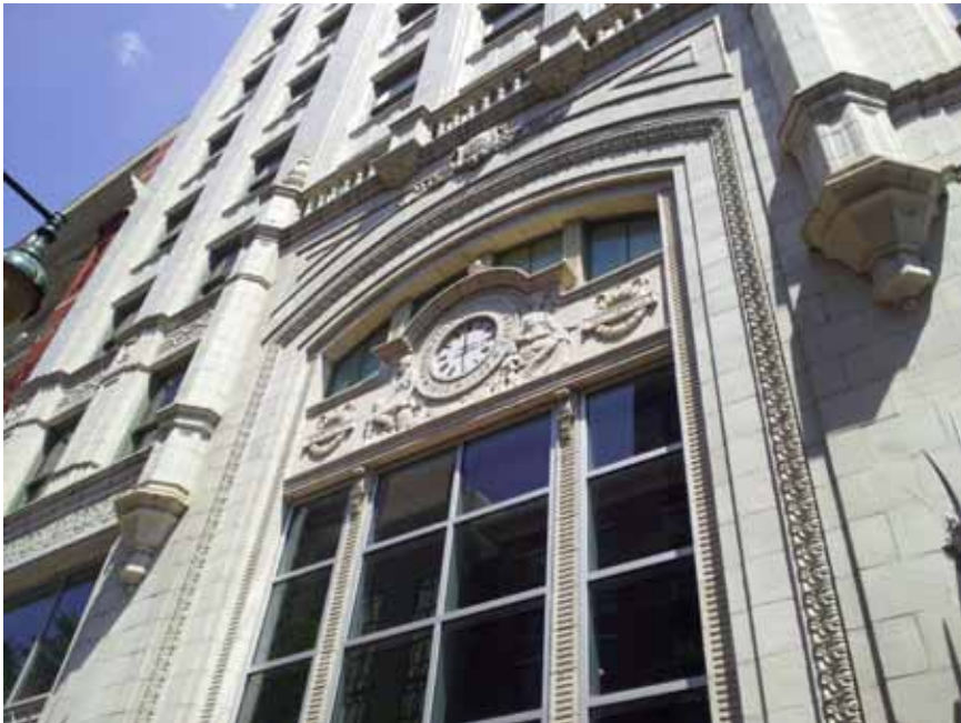
An example of architectural detailing that enhances the visual experience of the street.
