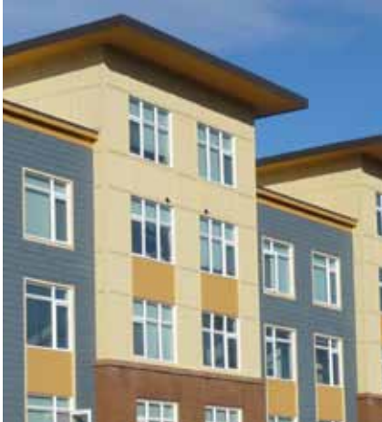
Fiber cement board, formed in lap siding or as a board and batten panel design, may be an appropriate material in residential areas.
