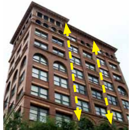
Provide vertical articulation in a larger building mass to establish a sense of scale.
