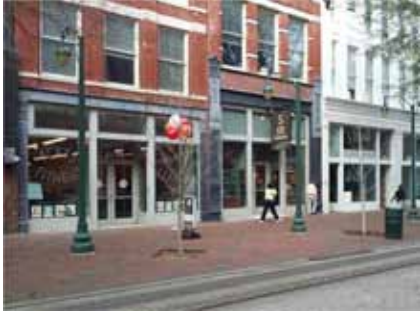
Windows, moldings, and transoms at the street level express the human scale of a building. Future development should relate to the proportions of these features and maintain the same sense of scale.
