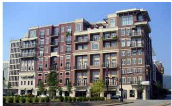
Variation in building height within a project contributes to sense of scale and creates a variegated skyline.
