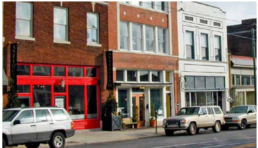
P6: Design for sustainability. Aspects of cultural, economic and environmental sustainability that relate to urban design and compatibility should be woven into all new improvements.
