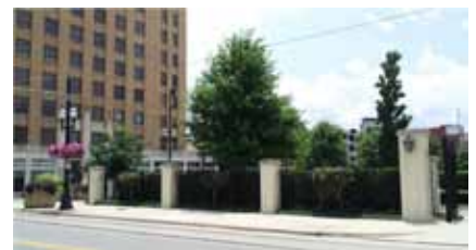
Where surface parking does exist, it should be screened with landscaping, fences, walls, or other decorative features.
