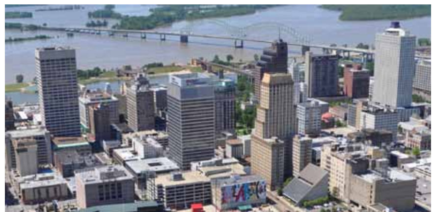
A new design should be compatible with traditional architecture in Downtown, but need not copy older styles.
