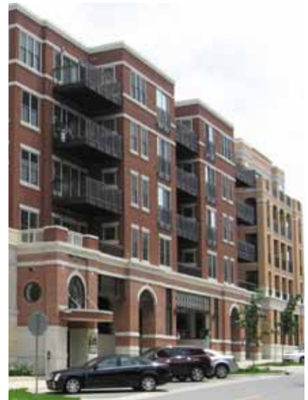
Use moldings, columns, a change in material or an offset in the wall plane to define different building modules.
