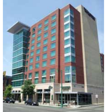
Variation in building height and massing is important to achieving a sense of scale.
