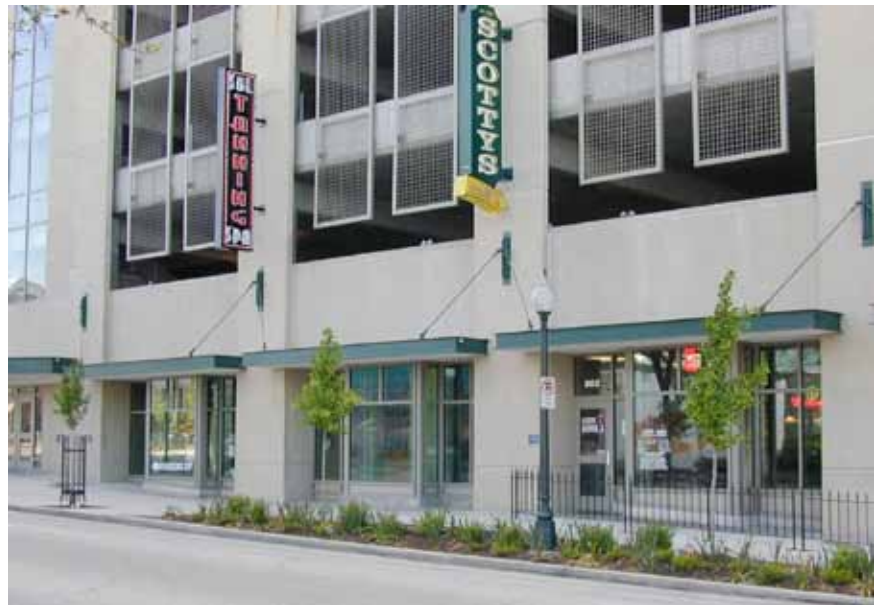
When parking in a structure occurs at the street level on a primary street, it shall have an active use at the sidewalk edge, as this one does.
