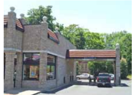
A drive-through facility should coordinate with the primary structure in terms of materials and architectural details.
