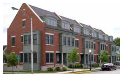
Use vertical and horizontal articulation design techniques to reduce the apparent scale of a larger building mass and to create visual interest. (Changes in materials, and projecting walls and balconies convey horizontal and vertical expression in these buildings.)
