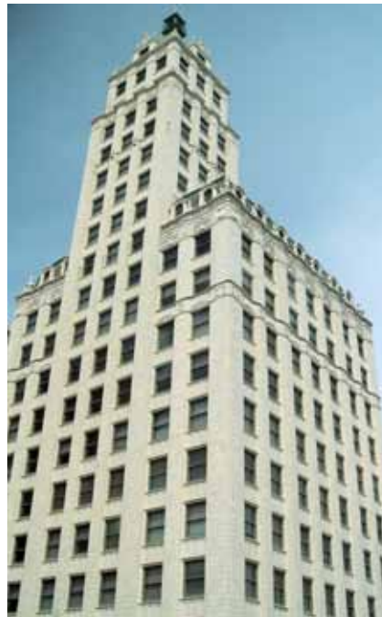
Provide variation in building height in a large project. (These examples illustrates historic precedent in Memphis for varying building height.)
