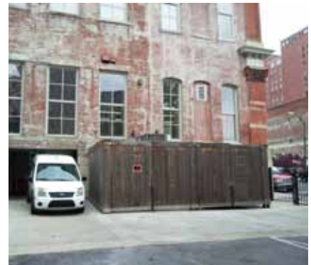
Mechanical units should ideally be located along the rear façade and screened from view.
