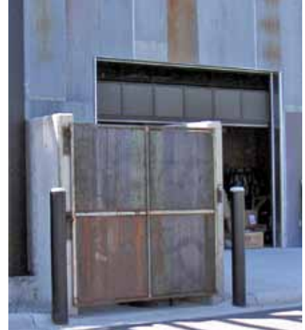
Screen equipment from view or design it to be visually subordinate to the building. (In this industrial context, a metal and concrete screen is used.)
