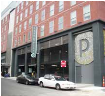
Complete screening of cars is not required, but it should be sufficient to minimize the visual impacts of autos.
