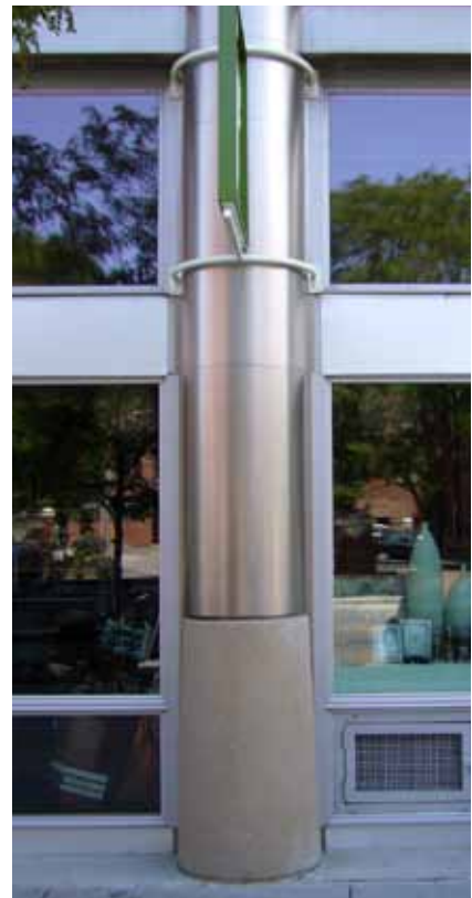
Projecting columns provide visual interest.
