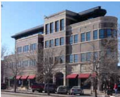
It is especially important in this context that the primary entrance of a building faces the street to help enhance the pedestrian-oriented environment.
