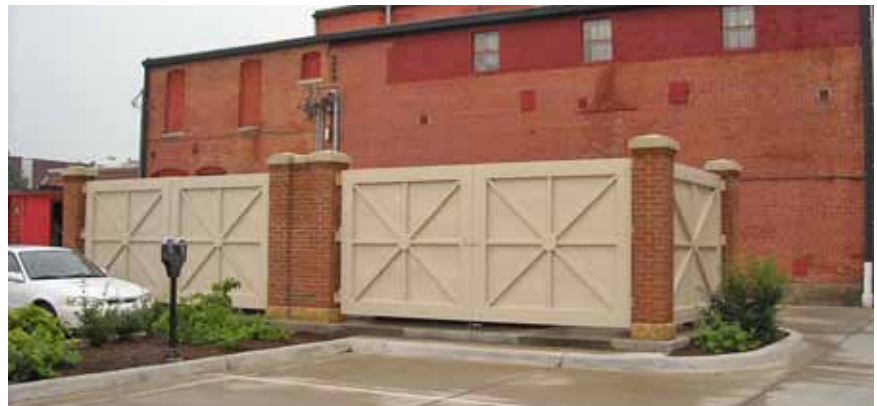
Service areas should be visually unobtrusive and should be integrated with the design of the site and the building, as this one is.
