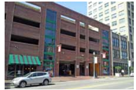
P13: Keep the automobile subordinate. Parking garages with ground floor uses engage pedestrians and mitigate the visual impact of parking areas.
