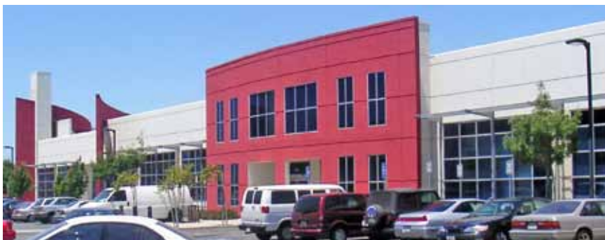
Use a change in design features to suggest the established range of building widths. (In this industrial context, variations in concrete modules convey scale.)
