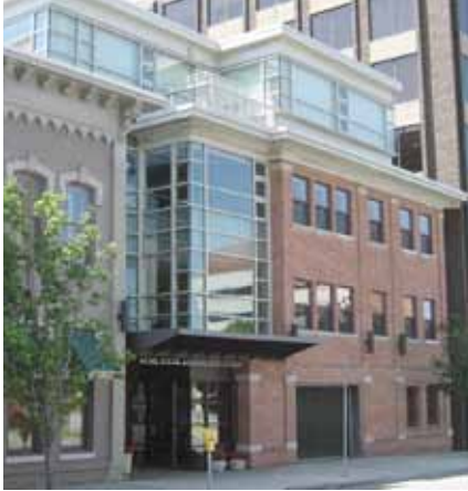
A new building should step down toward lower scaled neighbors, especially when adjacent to historic properties and edges of historic districts, as this one does.
