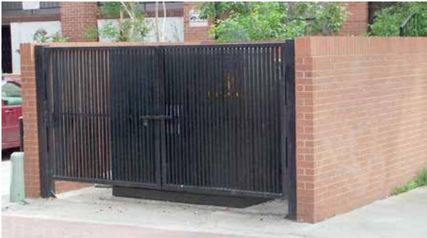
Screen equipment from view or design it to be visually subordinate to the building. (This screen uses materials that are similar to the primary building.)
