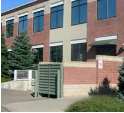
Screen a service area with a wall, fence or planting. (This brick wall is an example.)
