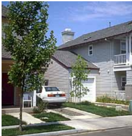
Consider using decorative and porous paving materials, and grass strips in driveways, as this driveway illustrates.
