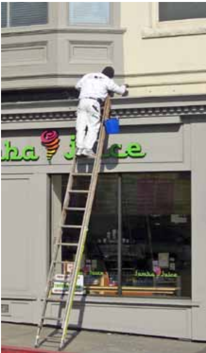
Repair deteriorated character-defining features.
