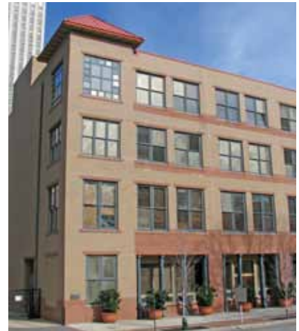
The first floor height should be taller than any upper floors and should appear similar in dimension to those seen traditionally.
