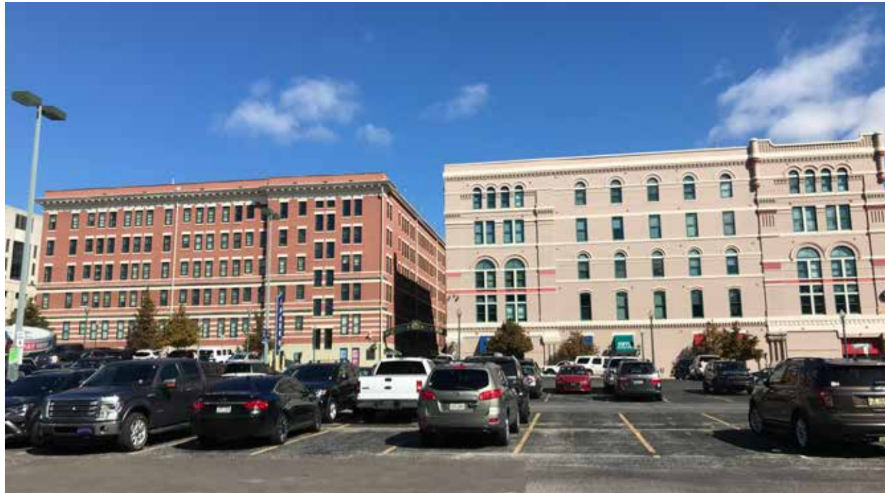
GAYOSO HOUSE, PEMBROKE SQUARE - PEABODY PLACE FAÇADE
