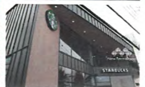
Wood siding with sheet metal siding
