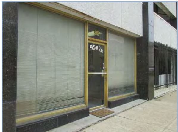
View showing the southeastern corner of the building, looking northwest
