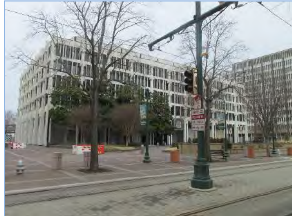
View of the northwestern surrounding property, looking northwest from the intersection of Adams Avenue and North Main Street
