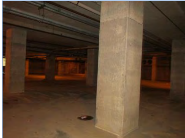
View of the parking garage
