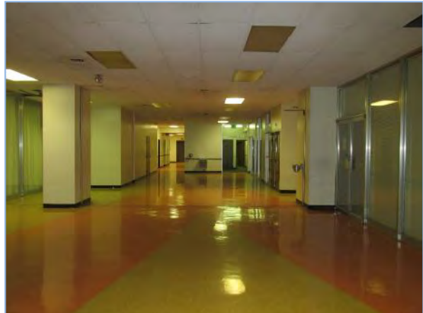
View of vinyl floor tile and acoustic ceiling tile within a common area lobby
