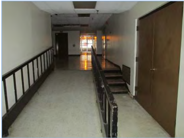
View of a typical hallway
