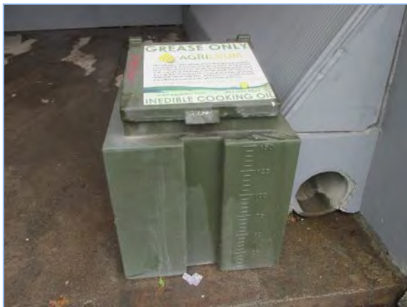
View of the waste kitchen grease container in the loading dock area
