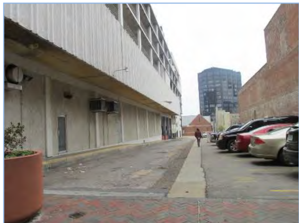
View along the southern side of the site building, looking east
