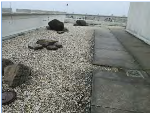
View of roofing and roof flashing materials
