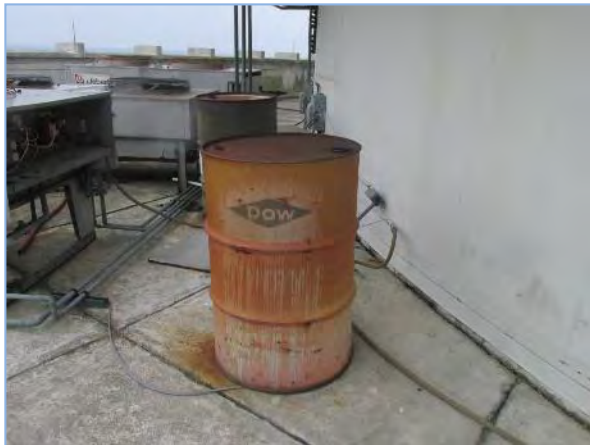
View of two drums located on the lower building roof
