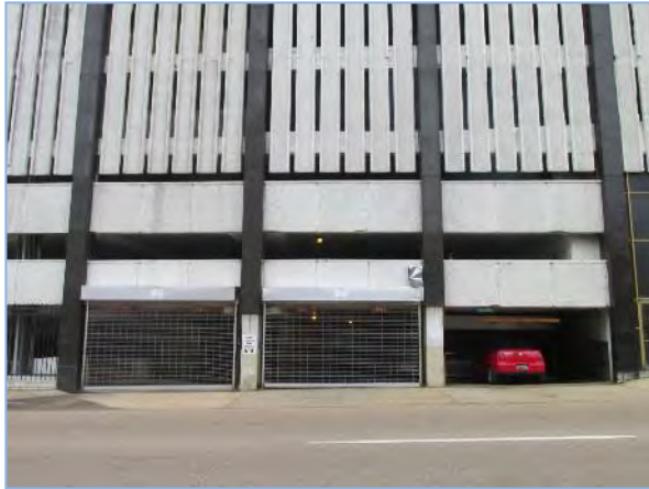
View showing the eastern side of the building, looking west
