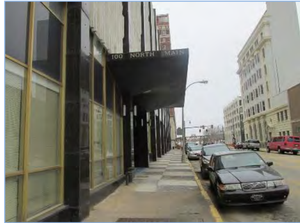
View along the northern side of the building, looking west
