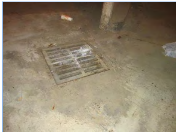
View of a typical parking garage storm drain
