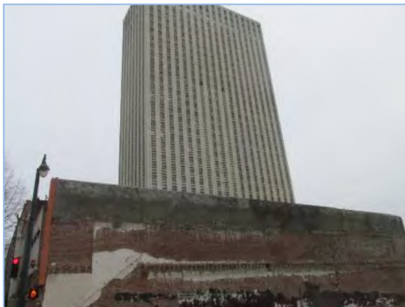
View of the site building, looking north from Jefferson Avenue
