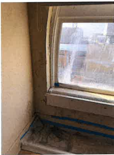
Images of current window conditions indicating need for full window replacement on floors 2 and 3
