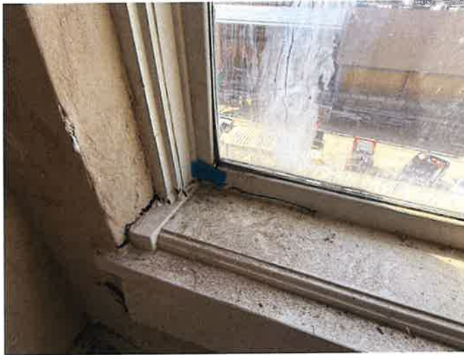
Images of current window conditions indicating need for full window replacement on floors 2 and 3
