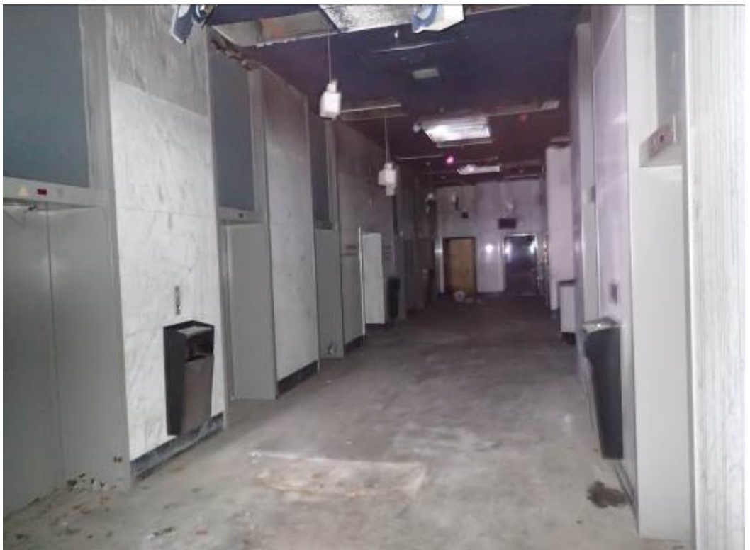
Photograph Number 10: View of foyer and elevators
