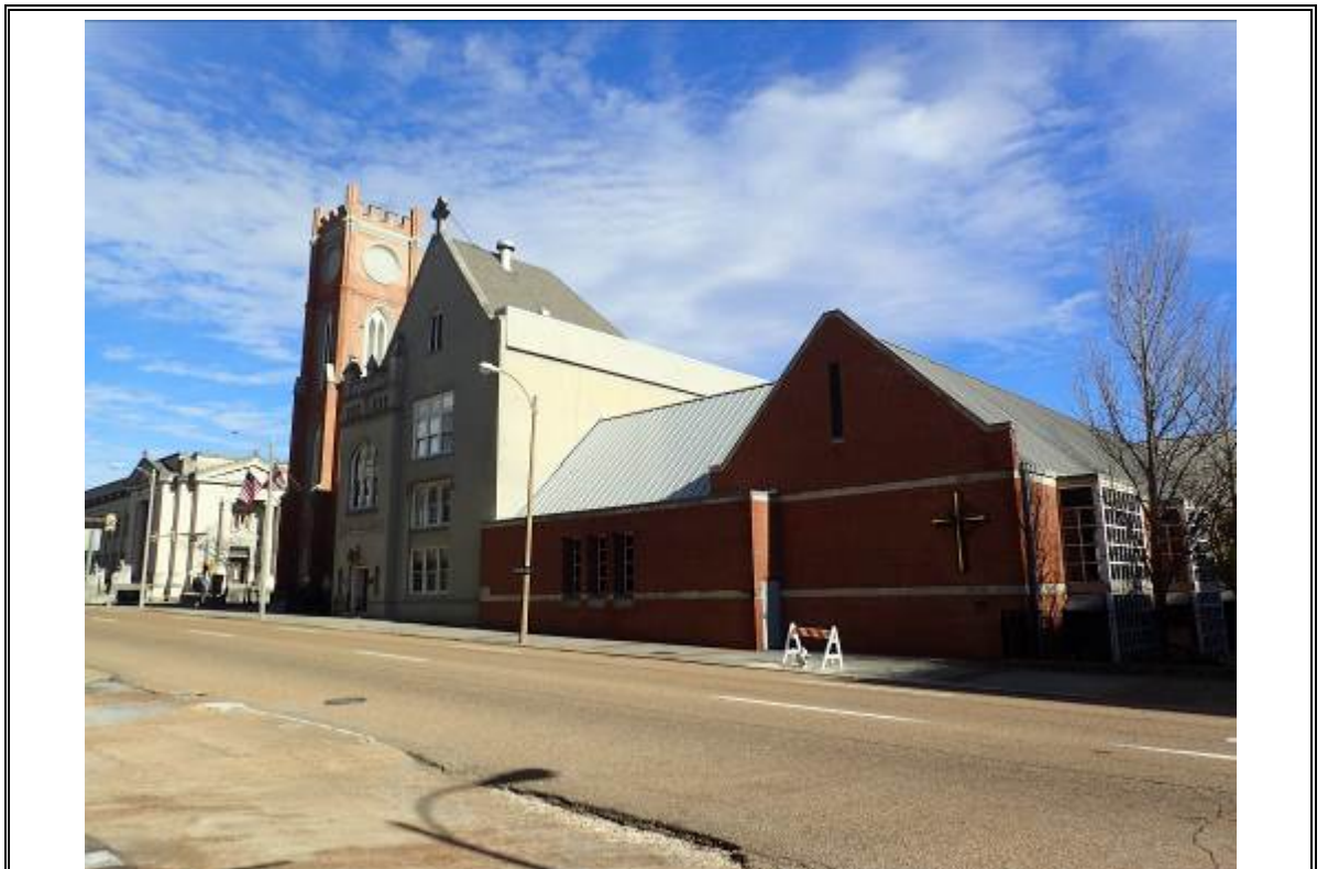
Photograph Number 16: View of adjacent properties to the east
