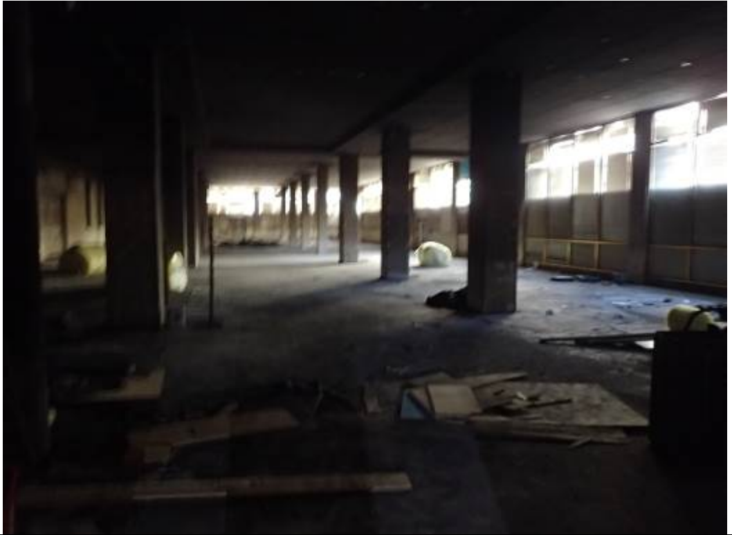
Photograph Number 9: View of parking garage
