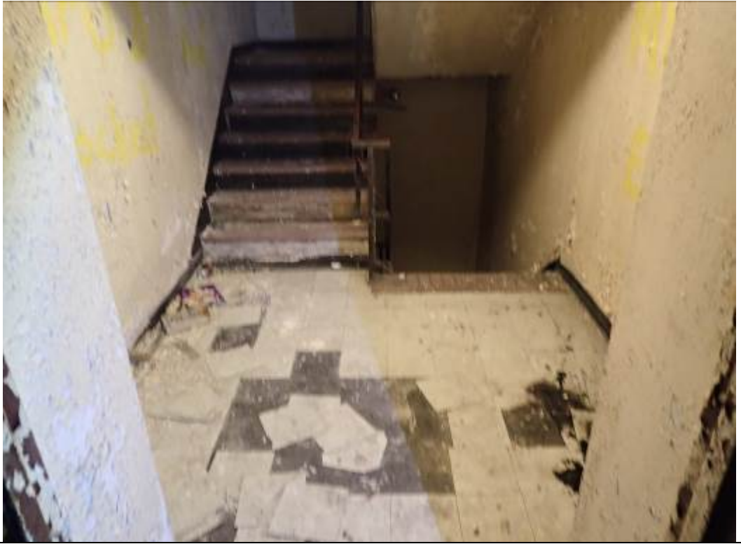
Photograph Number 11: View of stairwell
