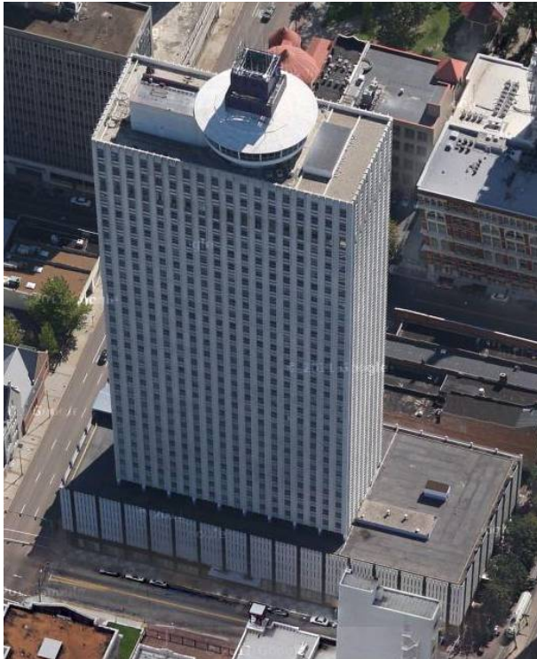
100 N Main Exterior
