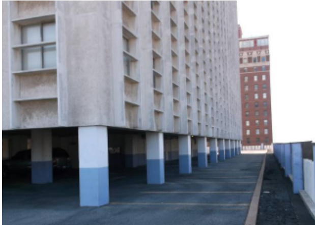
Base of Tower at 8 th Level Roof
