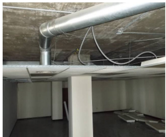
Typical Flat Slab at Interior Column
