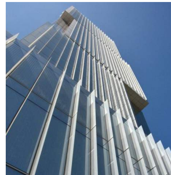
CURTAIN WALL WITH VERTICAL FINN ACCE- TUATING THE HEIGHT OF THE TOWER
