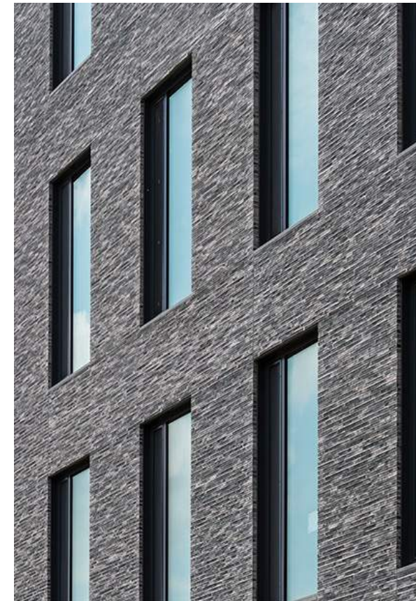
PUNCHED OPENINGS ON BRICK MASSING
