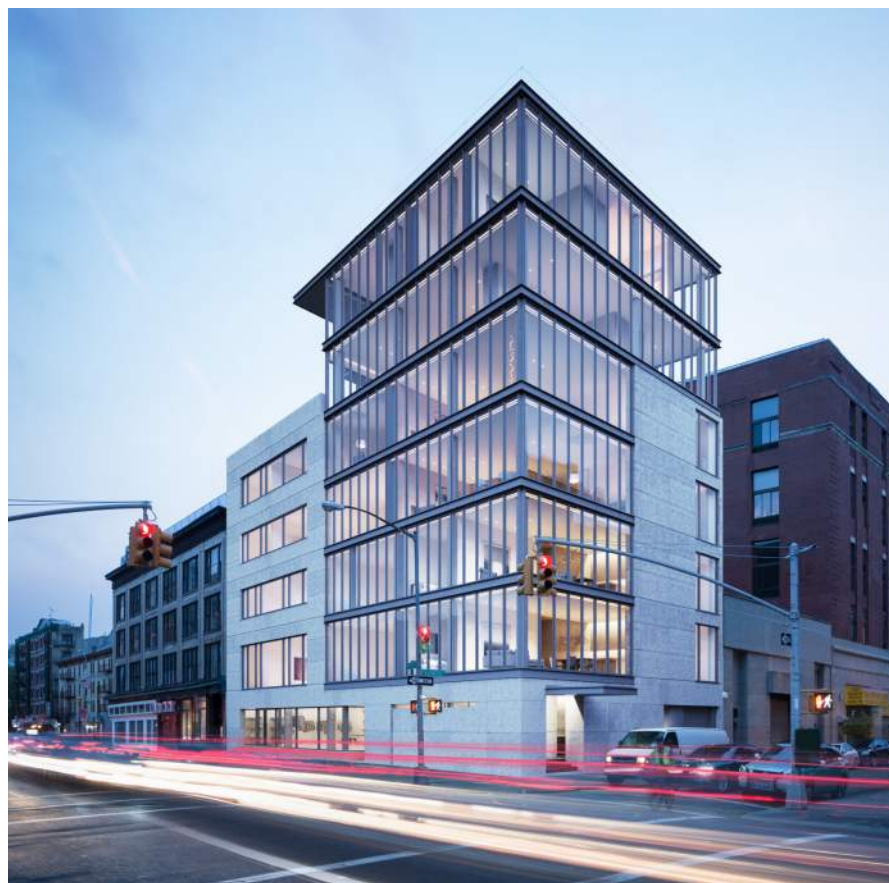
GLASS ENCLOSURE PROTRUDING OUT FROM THE WAREHOUSE
