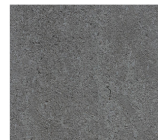
Concrete Base No Finish
