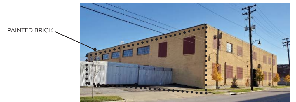
NORTH WEST CORNER
